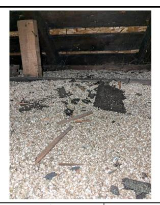
Material Description: Vermiculite Insulation – Tested Positive for Asbestos
