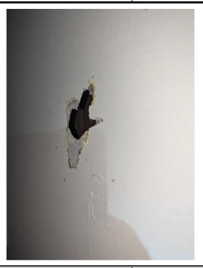
Material Description: Transite Wall - Tested Positive for Asbestos
