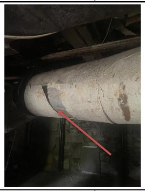
**Material Description:** Pipe Wrap - Tested **Positive for Asbestos**
