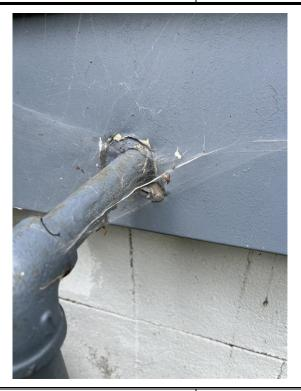
Material Description: Penetration Caulking-Tested Positive for Asbestos
