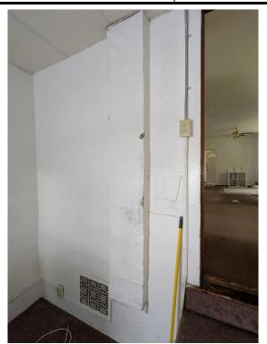
Material Description: Vent Insulation – Tested Positive for Asbestos
