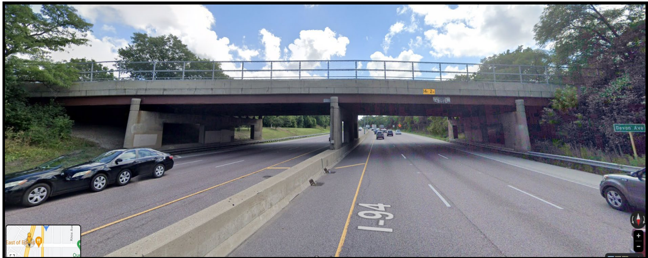
Exhibit 2 Devon Avenue over I-94 (Eastbound on I-94)
