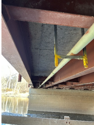
EXISTING GAS MAIN MOUNTED TO UNDERSIDE OF DEERFIELD ROAD BRIDGE OVER DES PLAINES RIVER
