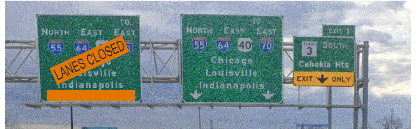
CONTRACTOR TO COVER "ARROWS" WITH ORANGE PLAQUE
