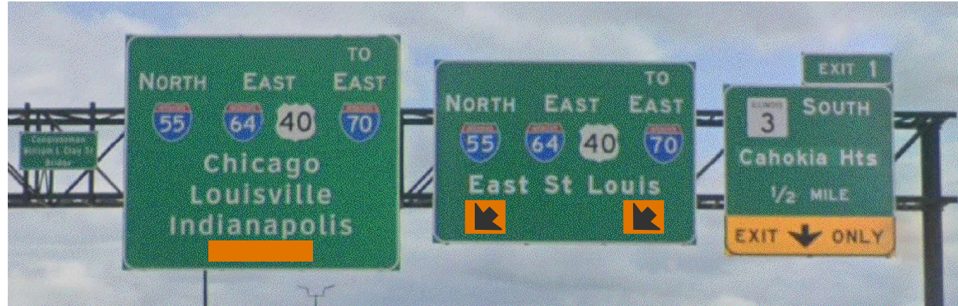
CONTRACTOR TO COVER "ALL LANES" TEXT WITH ORANGE PLAQUE
