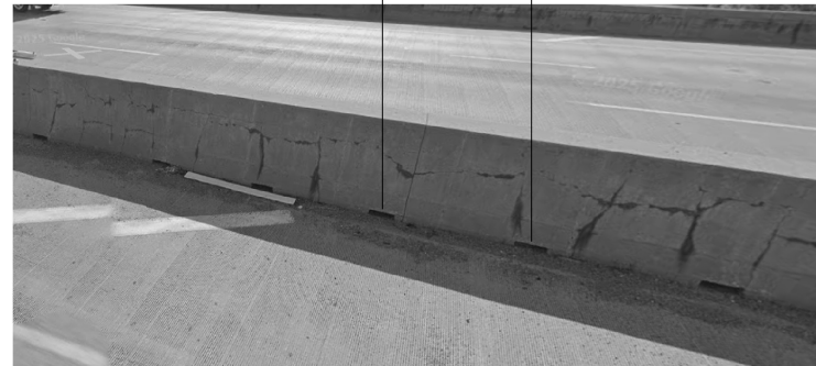
CAST OPENINGS IN MEDIAN BARRIER
