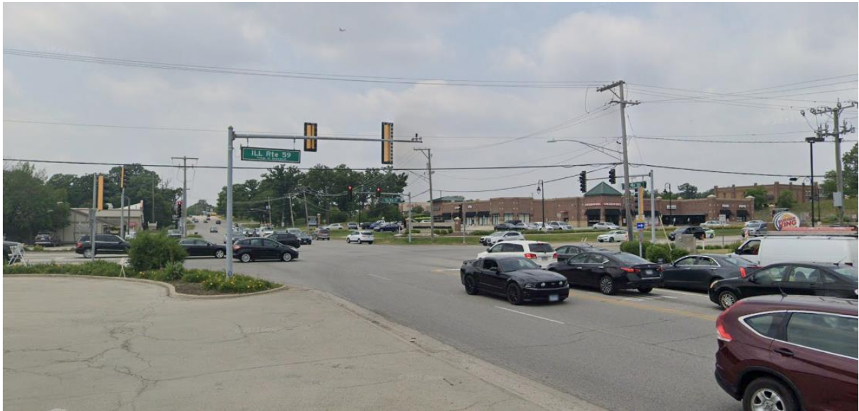
Existing signalized intersection of US 52 and IL 59 looking west. There is no roadway lighting provided except for some isolated beacon lights attached to ComEd utility poles.
