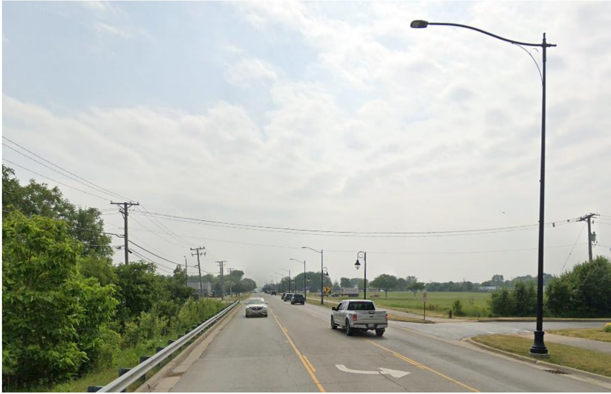
Existing Village of Shorewood ornamental lighting along US 52 east of River Road showing separate poles for roadway and pedestrian luminaires.
