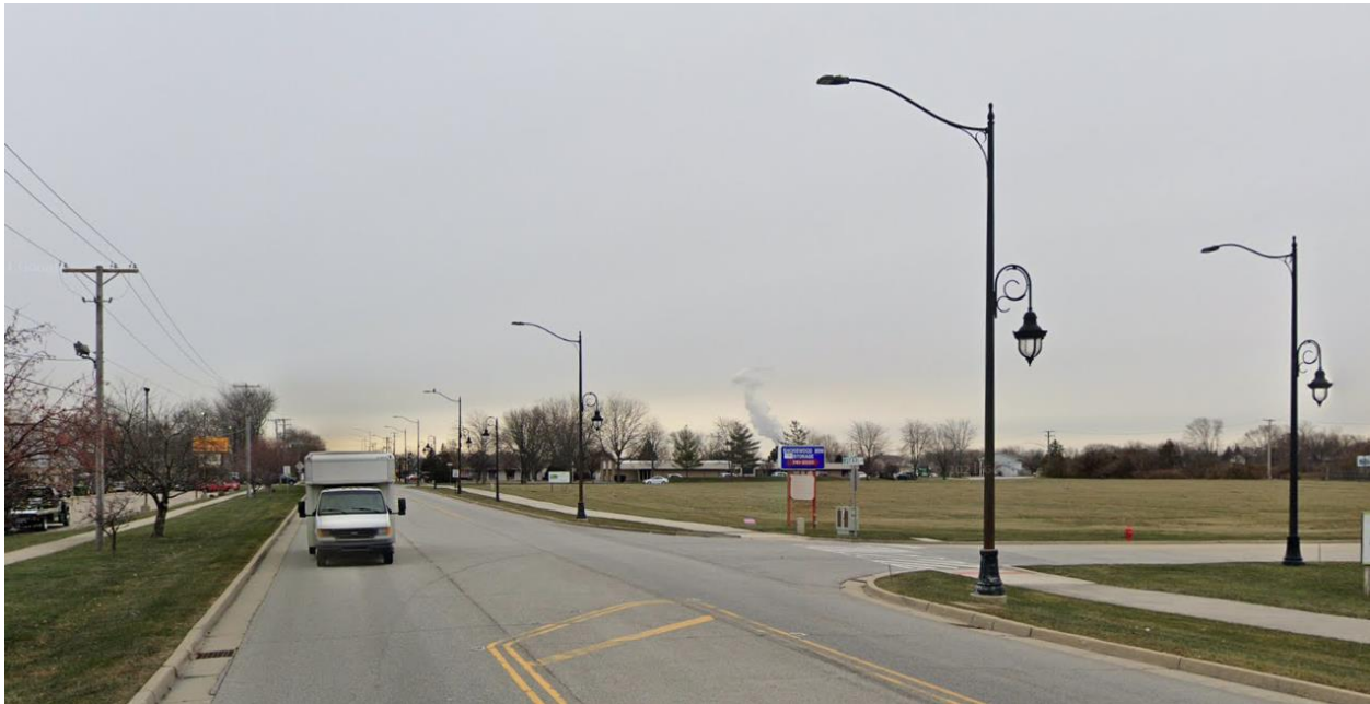
Existing Village of Shorewood Ornamental lighting along US 52 at Earl Drive showing roadway poles with “piggy back” pedestrian luminaires.
