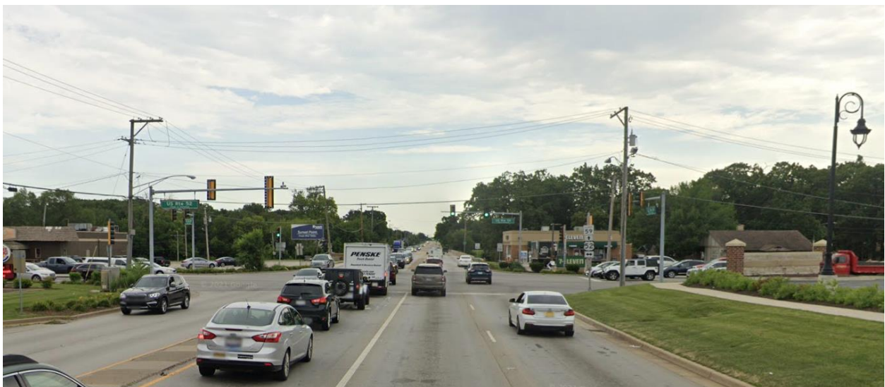
Existing signalized intersection of US 52 and IL 59 looking south. There is no roadway lighting provided except for some isolated beacon lights attached to ComEd utility poles. Note the ornamental fixture shown on the right side of the photo belongs to a private development located on the northwest corner of the intersection.
