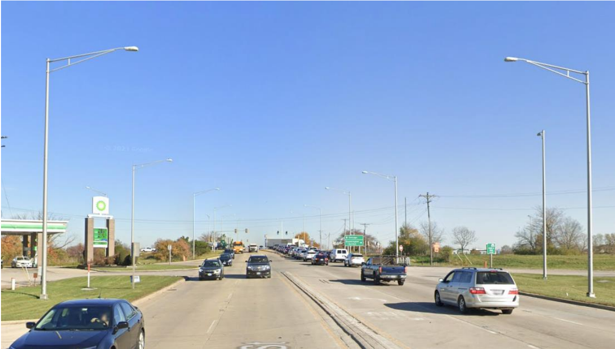
Existing IDOT interchange lighting along US 52 at West Frontage Road (looking east).
