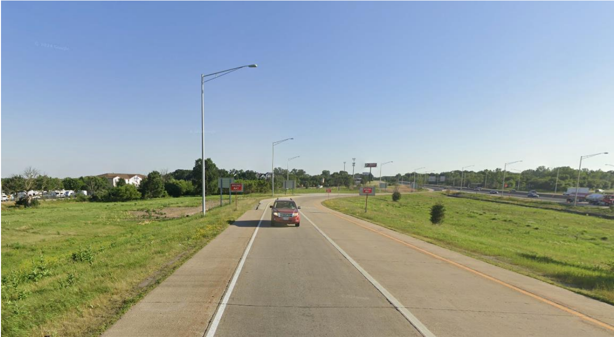
Existing IDOT interchange lighting along I-55 Ramps at US 52 (typical).
