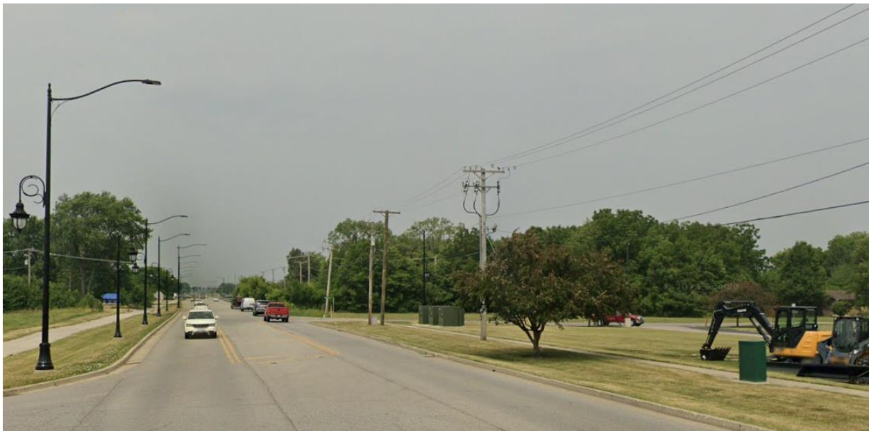
US 52 looking west at Earl Drive intersection. Existing Village of Shorewood ornamental lighting system controller is located on the north parkway of US 52 across from Earl Drive (lower right of the photo).
