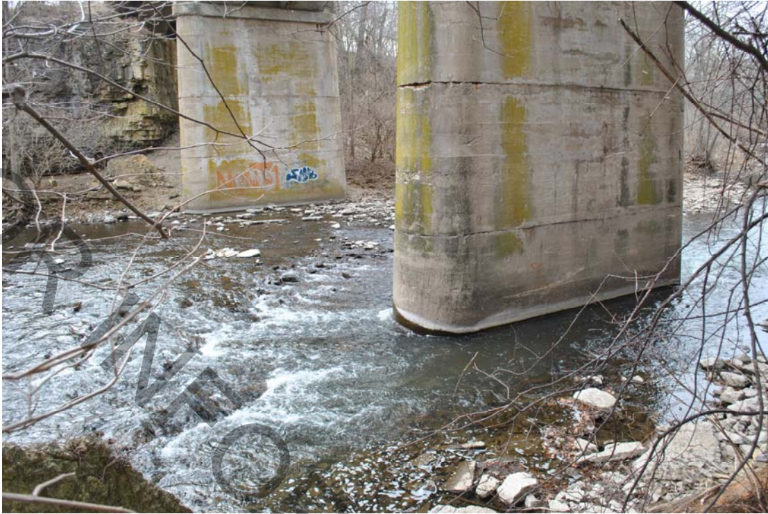
Figure 6: Image of creek bottom at IL 102 Bridge SN 046-0065
