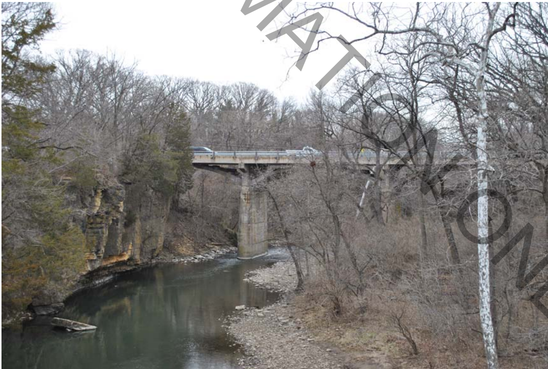
Figure 7: Image of existing structure SN 046-0065 from foot bridge downstream.
