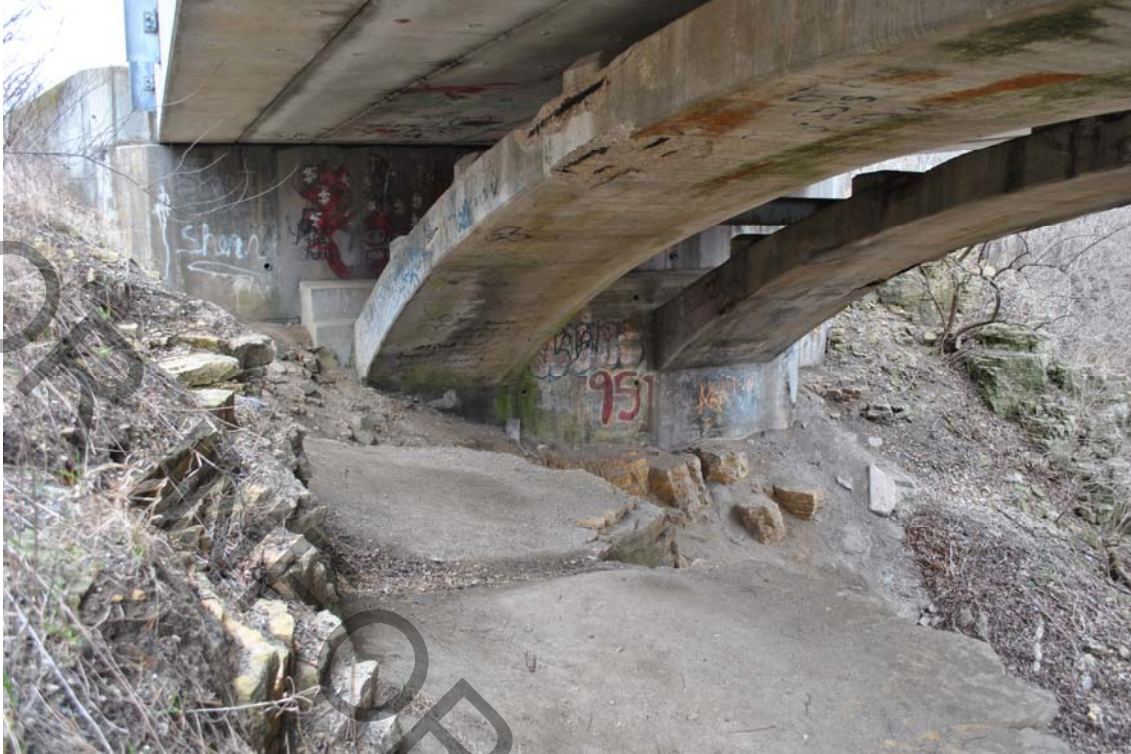
Figure 8: Existing east abutment.
