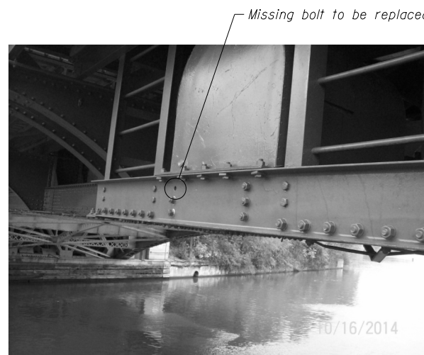
PHOTO 16: SOUTH MECHANICAL PLATFORM (Between Floorbeams 7 and 8 - EAST LEAF)
