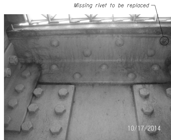
PHOTO 10: FLOORBEAM 4 TOP FLANGE (East Face of Floorbeam 4 - WEST LEAF)
