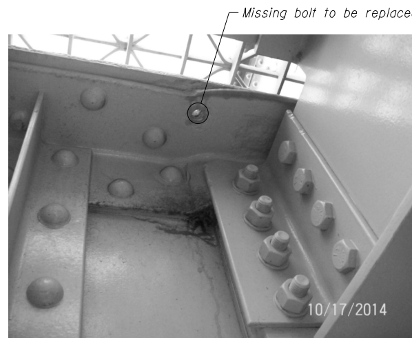
PHOTO 11: STRINGER 17 CONNECTION AT FLOORBEAM 7 (South Truss - WEST LEAF)
