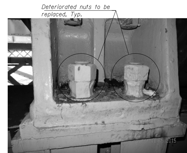
PHOTO 7: TRUNNION GIRDER BEARING DETERIORATED NUTS (Northeast Bearing - EAST LEAF)
