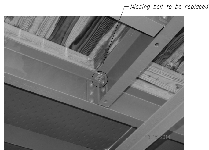
PHOTO 5: NORTH SIDEWALK STRINGER (Between Floorbeams 7 and 8 - EAST LEAF)
