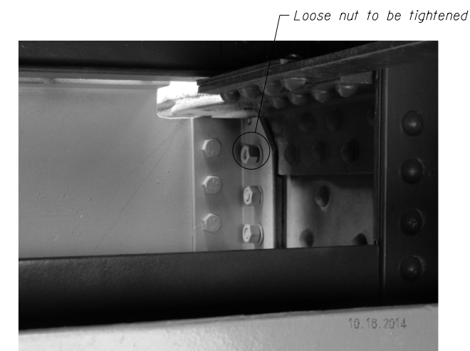
PHOTO 6: STRINGER 1 CONNECTION AT FLOORBEAM 7 (East Face of Floorbeam 7 - EAST LEAF)
