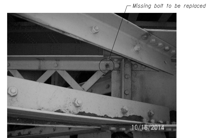
PHOTO 9: FLOORBEAM 2 BRACING CONNECTION (East Face of Floorbeam 2 - WEST LEAF)
