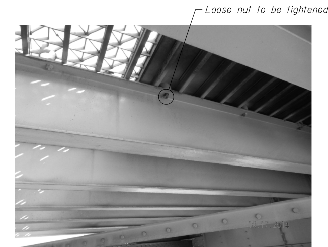
PHOTO 12: STRINGER 6 TOP FLANGE (Between Floorbeams 7 and 8 - WEST LEAF)
