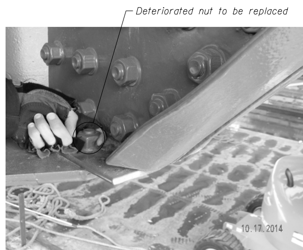
PHOTO 4: FLOORBEAM 7 NORTH BRACKET (North Truss - WEST LEAF)
