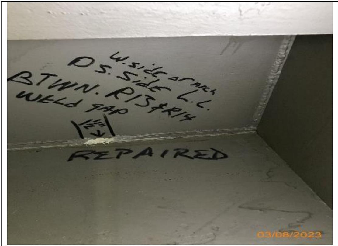
PHOTO 176 (Photo mislabeled, weld is not repaired.)
