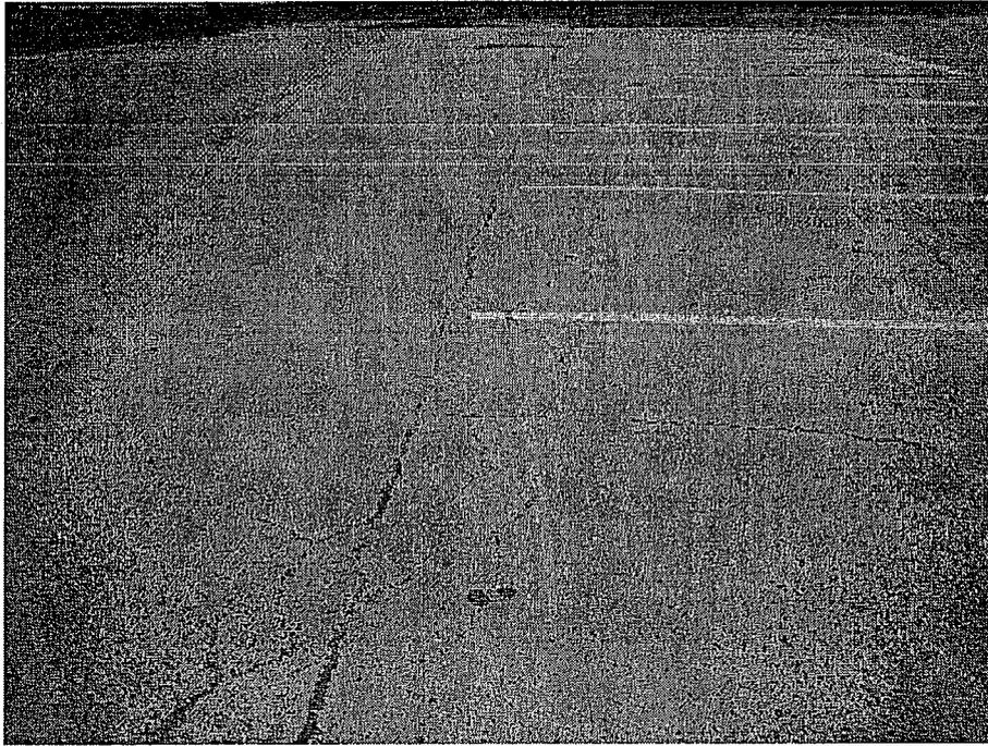
**Photograph 9: Facing south in southwestern parking area, moderate severity joint separation with spalled interconnected cracks.**
