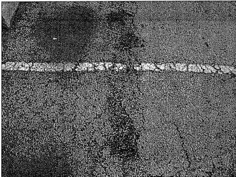
**Photograph 4: Raveling in eastern parking area with loss of fine and coarse aggregate.**
