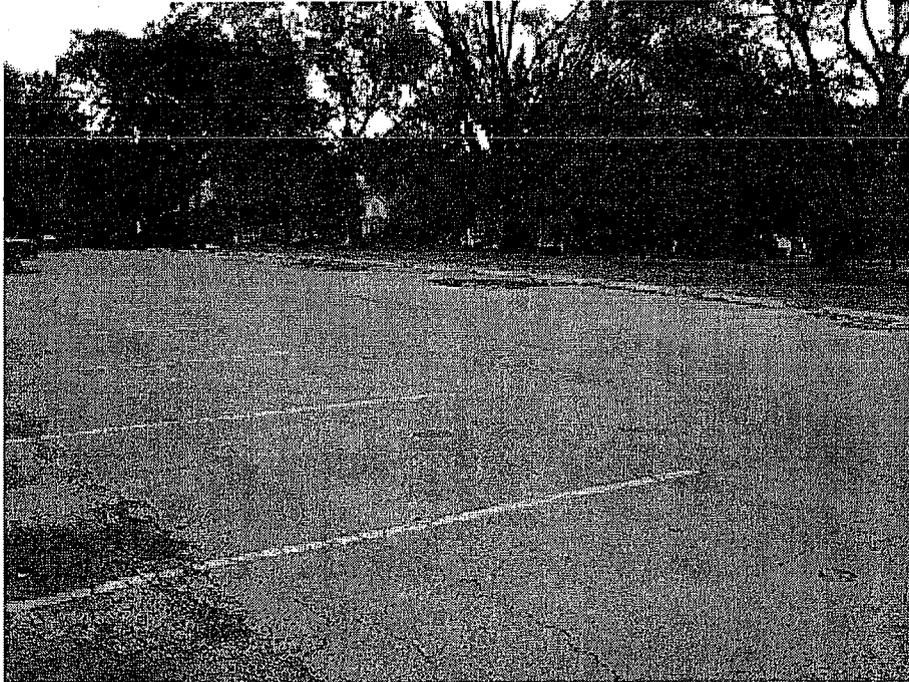
**Photograph 3: Facing southeast in eastern parking area, high severity fatigue cracking with spalled interconnected cracks and high severity raveling.**
