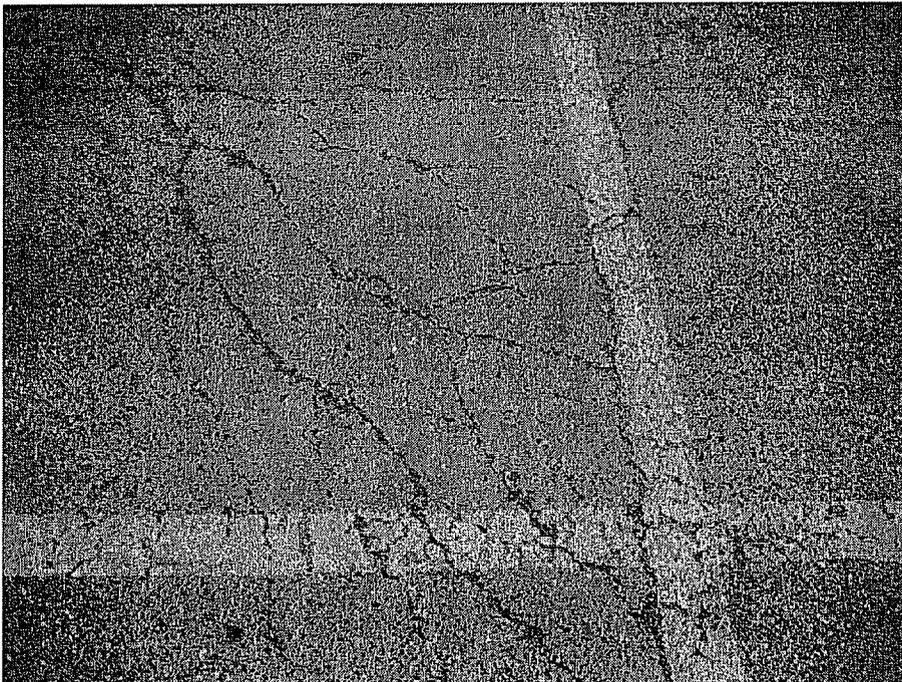
**Photograph 8: Close up view of moderate severity fatigue cracking with spalled interconnected cracks located within southwestern parking area.**
