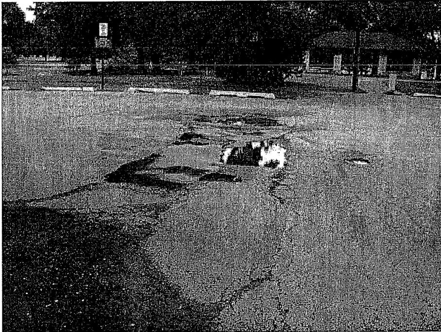
**Photograph 1: Facing west in eastern most parking area, high severity patch deterioration with spalled interconnected cracks.**
