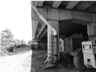
PIER 2 - EAST END (Looking South)
