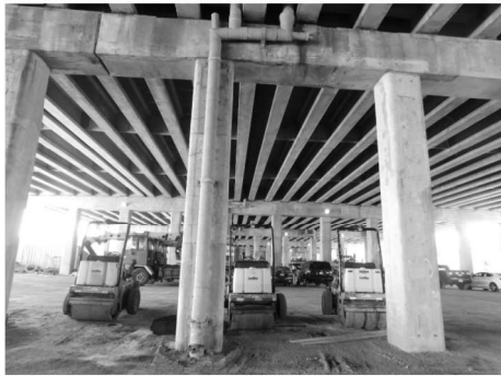
PIER 7 - WEST END (Looking South)
