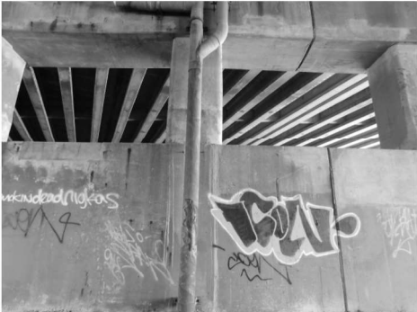
PIER 10- WEST END (Looking North)
