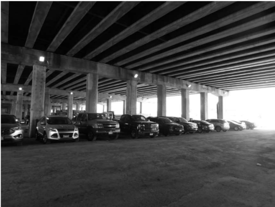
PIER 5 (Looking Northeast)
