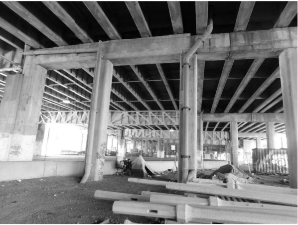
PIER 15 - WEST END (Looking North)
