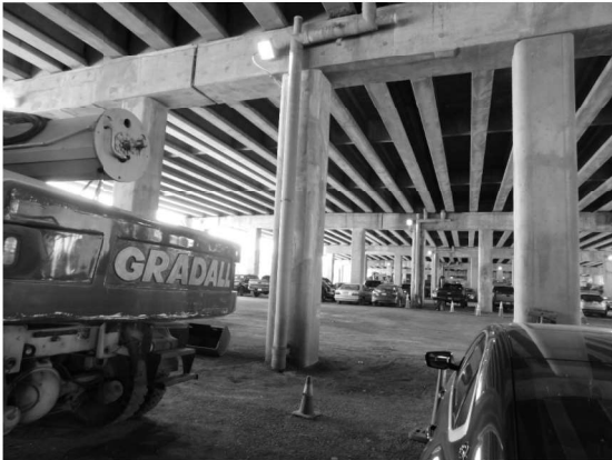
PIER 6 - WEST END (Looking South)
