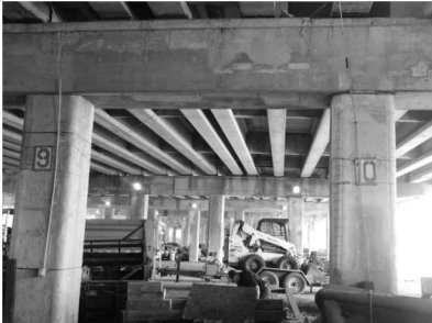
PIER 2 (Looking North)
