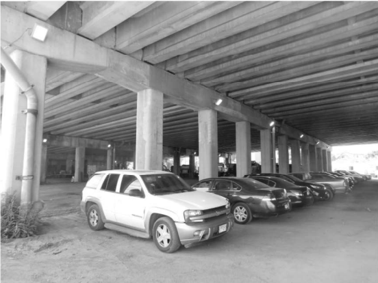
PIER 4 (Looking South)
