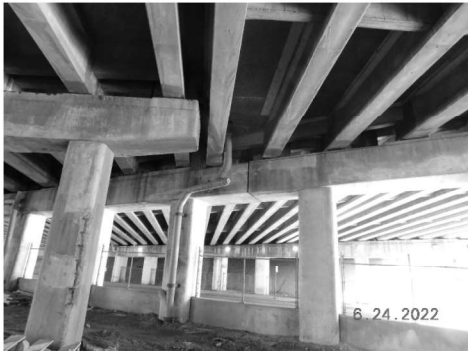
PIER 23 - WEST END (Looking North)
