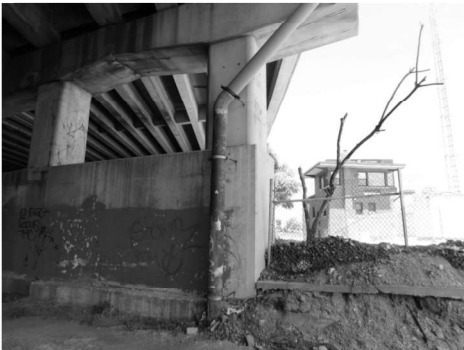
PIER 10 - EAST END (Looking North)
