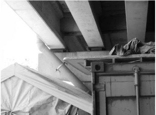
PIER 1 - EAST END (Looking South)
