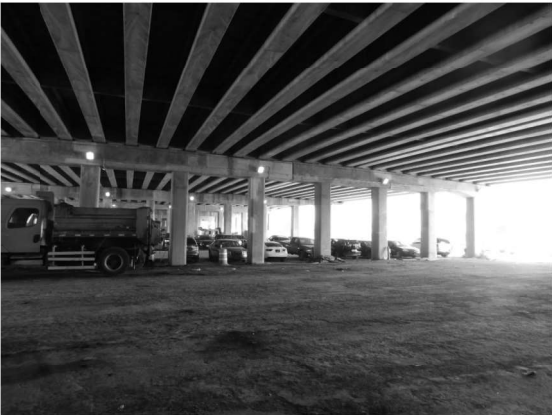
PIER 4 (Looking North)
