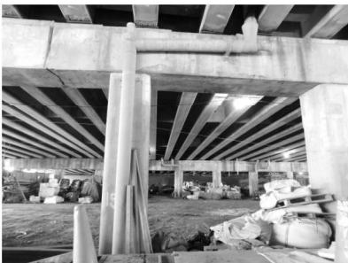
PIER 2 - WEST END (Looking South)
