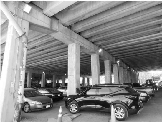
PIER 5 (Looking Southwest)
