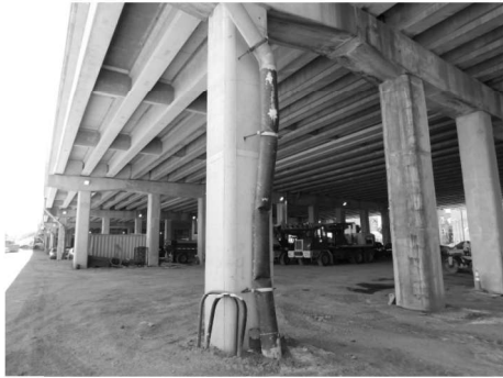
PIER 7 - EAST END (Looking Southwest)
