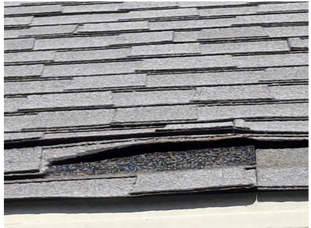
HA-37: Black Asphalt Shingle (Garage) HA-38: Tar Paper Layer under HA-37 (Garage)
