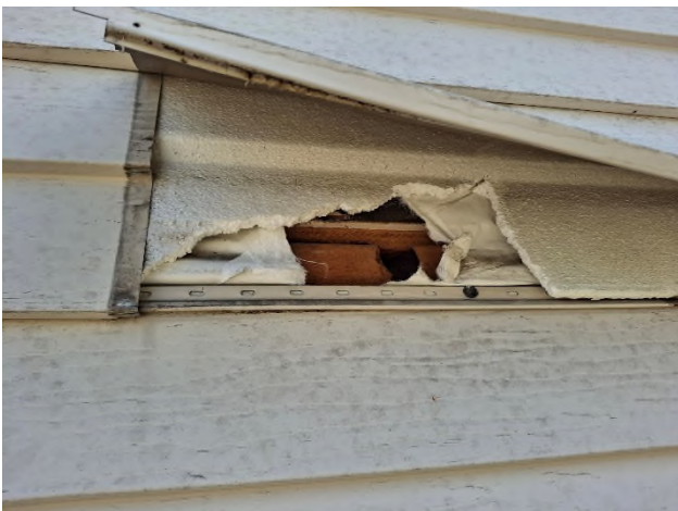
HA-39: White Vapor Barrier beneath Vinyl Siding
