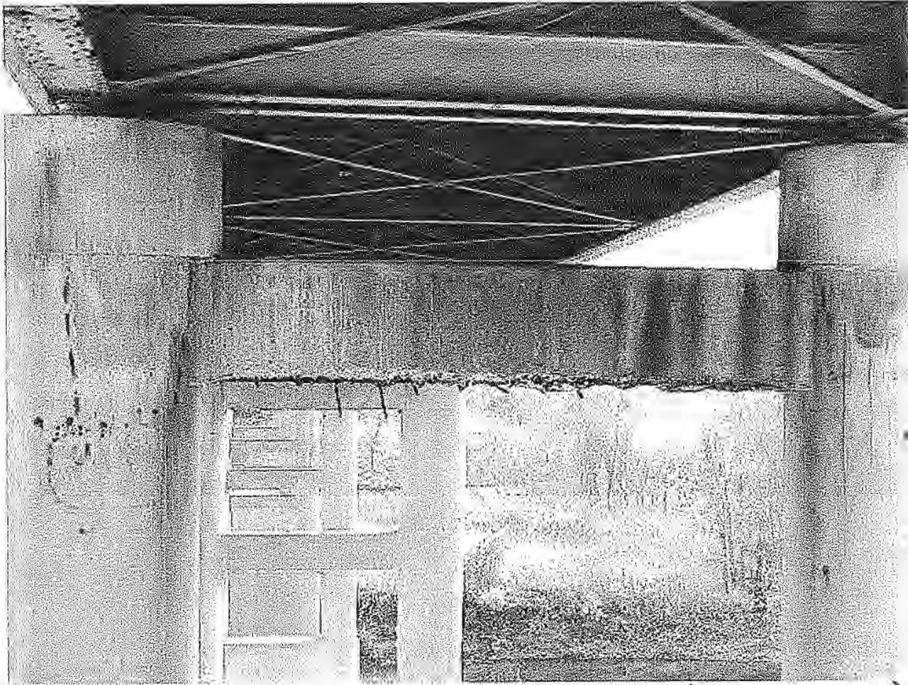
Pier 1A deterioration (TOP PIED DIA)
