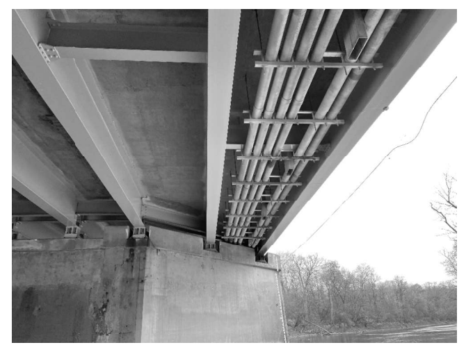
EXISTING UTILITIES BETWEEN BEAMS 5 AND 6
