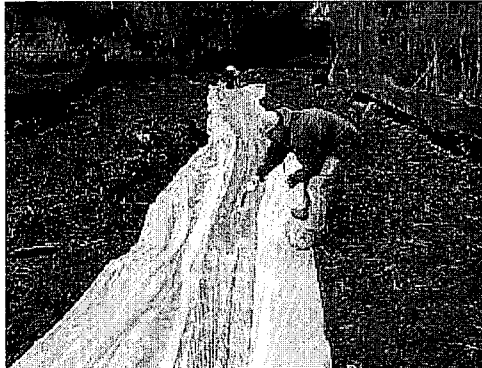
5) Apply Silt Stop (downstream end)
