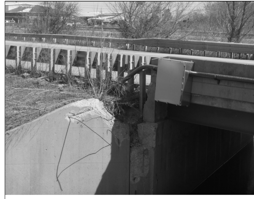
NORTH WEST CONCRETE WING WALL REPAIR (S.N. 099-0010)
