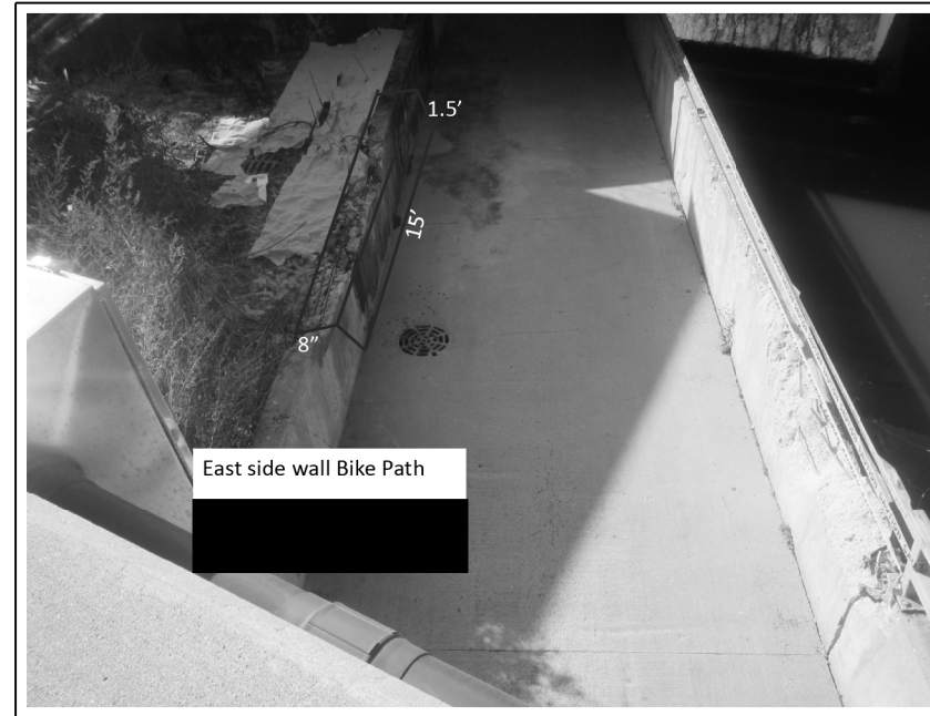
LOCATION 15 B BIKE PATH EAST SIDE CONCRETE WALL REPAIR-22.5 SQ. FT
