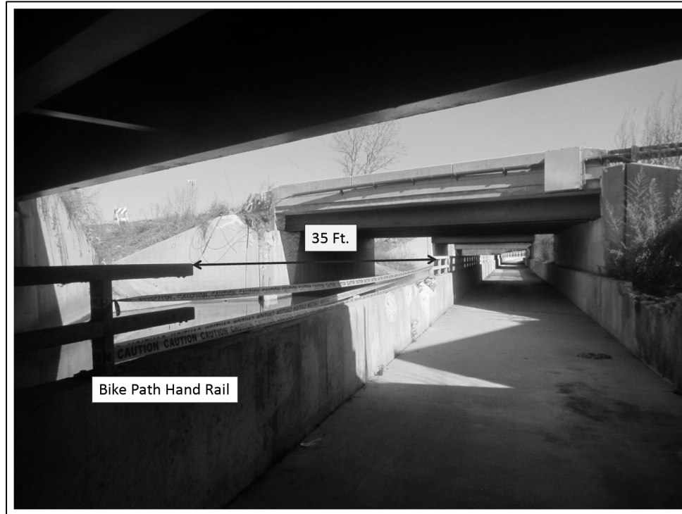
LOCATION 15 B PLACE 35 FT OF STEEL RAILING S-1
