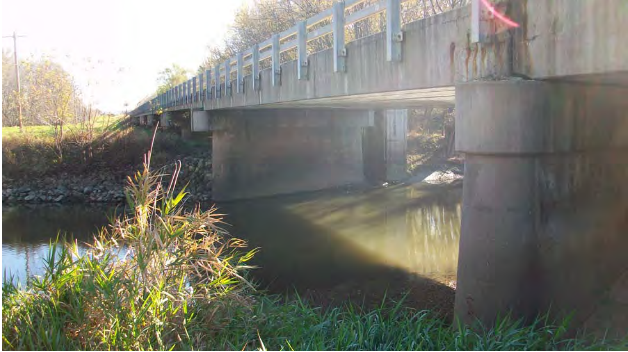
Photo 5 North Side of River Crossing
