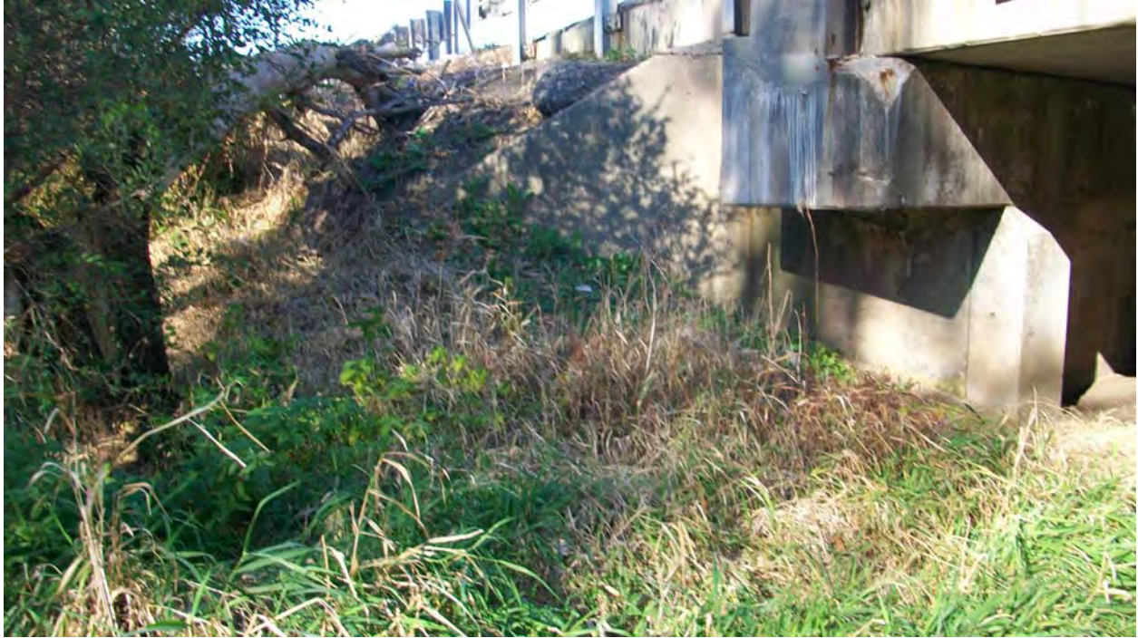
Photo 7 West Abutment Slope – North Side
