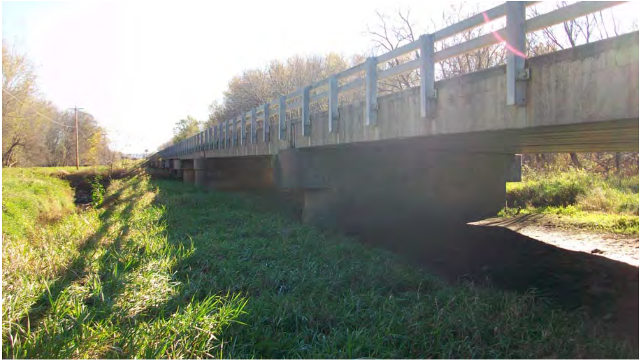
Photo 3 Looking East from West End – North Side
