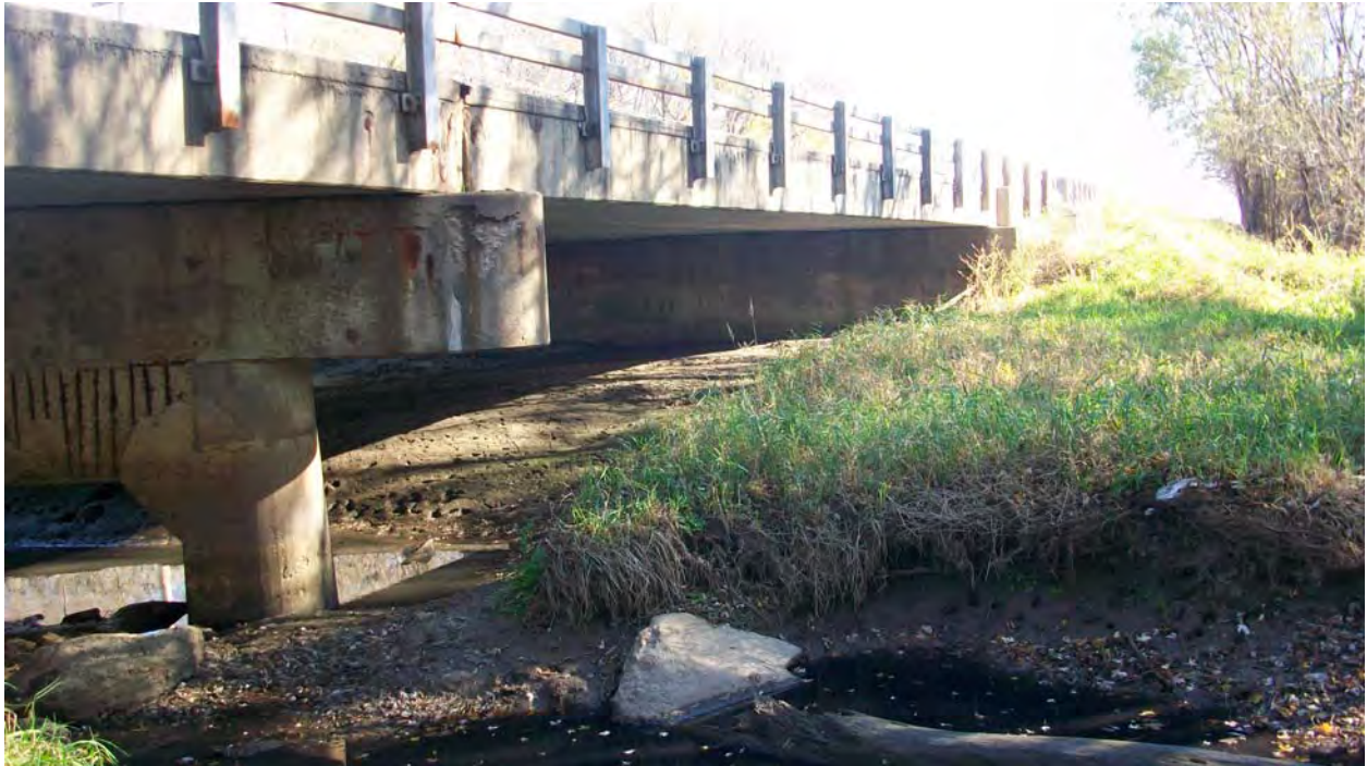
Photo 1 East Abutment Slope – South Side
