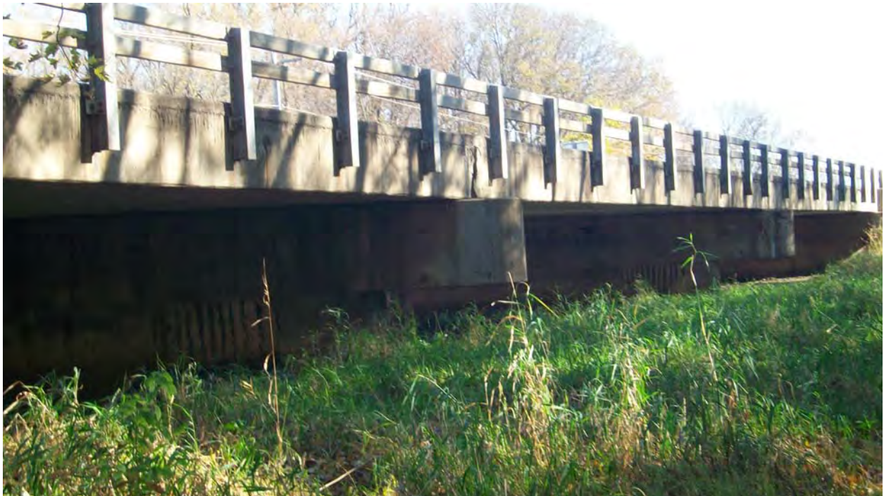
Photo 2 Looking East from River – South Side
