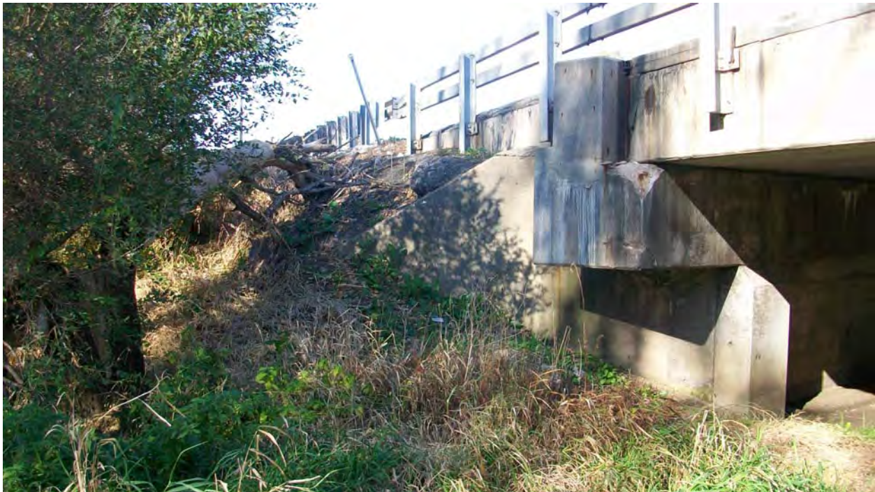
Photo 6 West Abutment Slope – South Side
