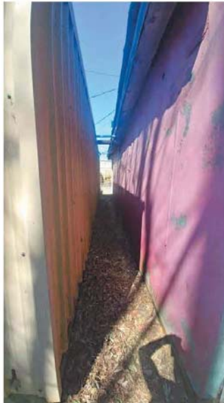
Old Maintenance – South Face & Aerosol Building – North Face
