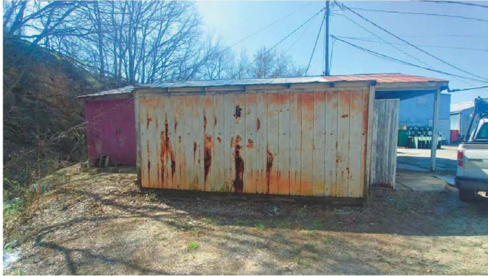
Old Maintenance - North Face
