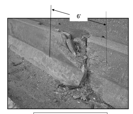
FULL DEPTH REPAIR REPLACE 6 FT OF BARRIER WALL FOR MORE DETAILS SEE SHEET # 8
