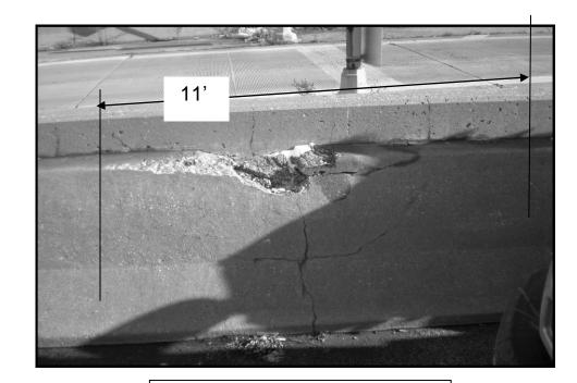
**FULL DEPTH REPAIR** REPLACE 11 FT OF BARRIER WALL FOR MORE DETAILS SEE SHEET #8
