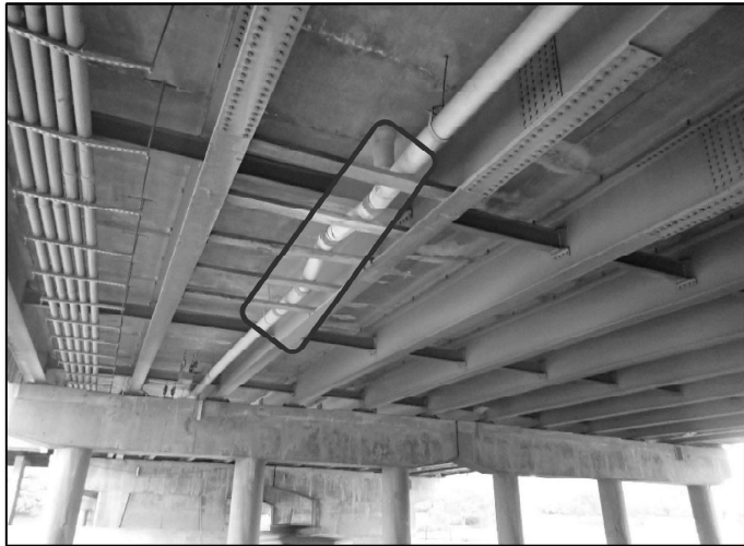
016-1160 PHOTO #1 NORTH SIDE OF BRIDGE OVER S.B. LOCALS REPLACE LONGITUDINAL SECTION (NORTH SIDE OF BRIDGE OVER S.B. LOCALS), 24 FEET
