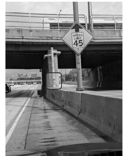
016-0189 PHOTO #1 PIER 4 SOUTH NOSE REPLACE SHORT SECTION ABOVE BARRIER WALL, 4 FEET
