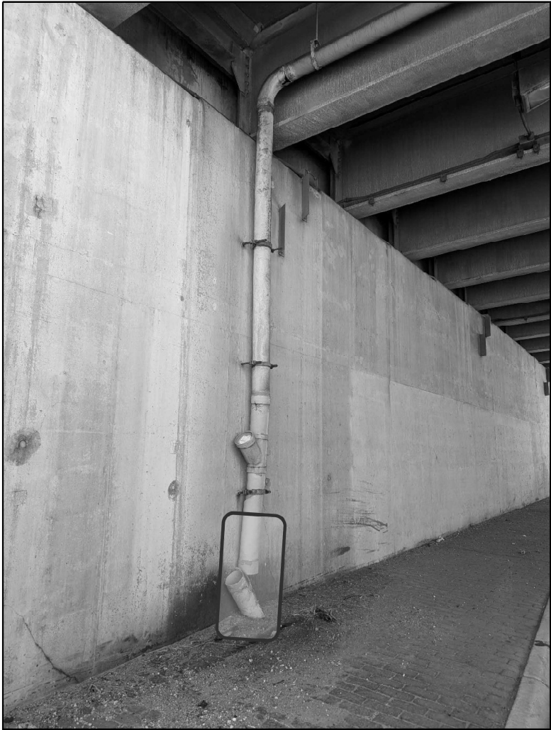
016-2850 PHOTO #1 EAST ABUTMENT - NORTH SIDE OF BRIDGE REPLACE BOTTOM OF PIPE, 4 FEET
