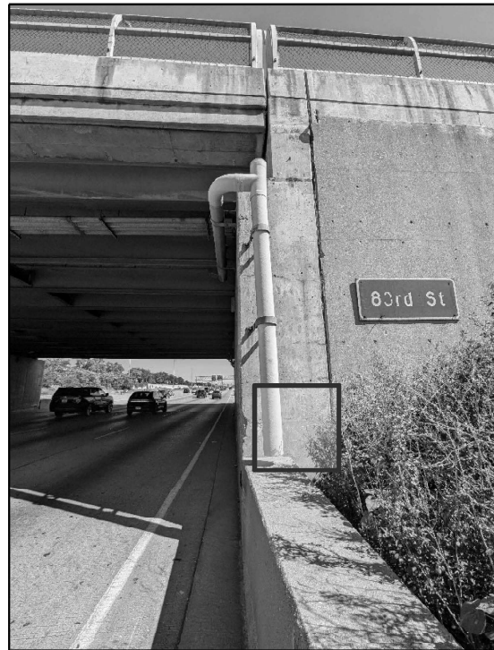
016-1143 PHOTO #3 EAST ABUTMENT - SOUTH END ELBOW TO PUSH WATER BEHIND BARRIER, 4 FEET
