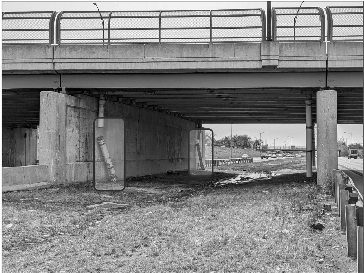
016-0989 PHOTO #1 CENTER MEDIAN - WEST FACE OF EAST PIER REPAIR BOTTOM SECTIONS OF BOTH DOWNSPOUTS, 24 FEET
