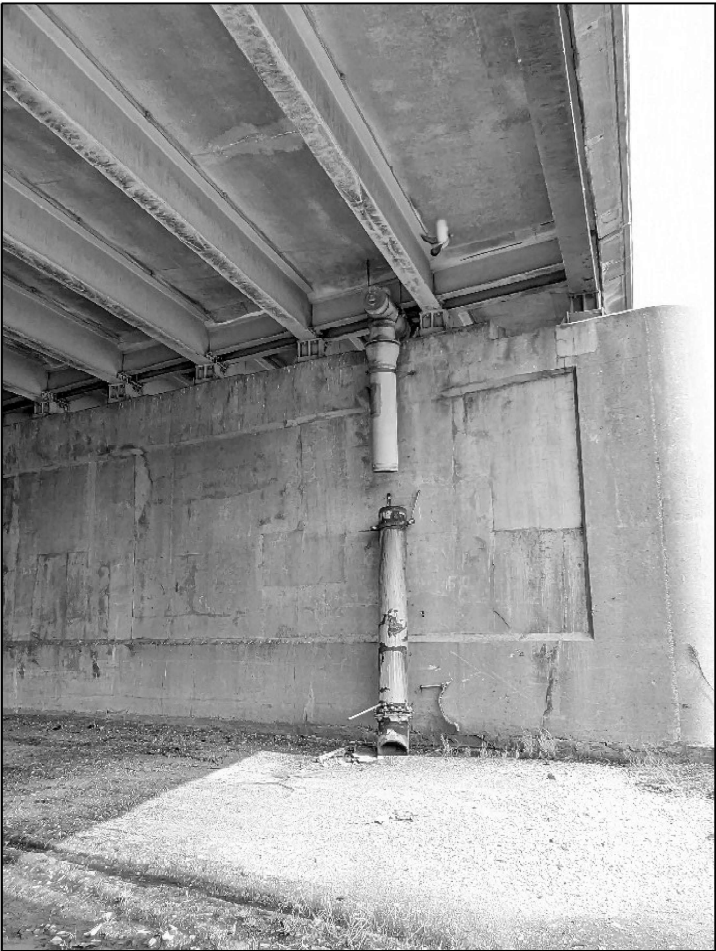
016-0989 PHOTO #3 WEST FACE OF EAST PIER - SOUTH PIPE
