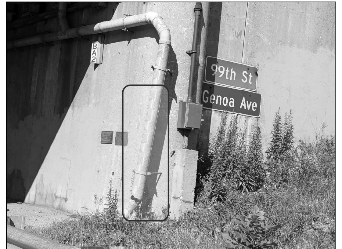
016-2030 PHOTO #1 NORTHWEST CORNER OF BRIDGE REPLACE BOTTOM SECTION OF PIPE, 8 FEET
