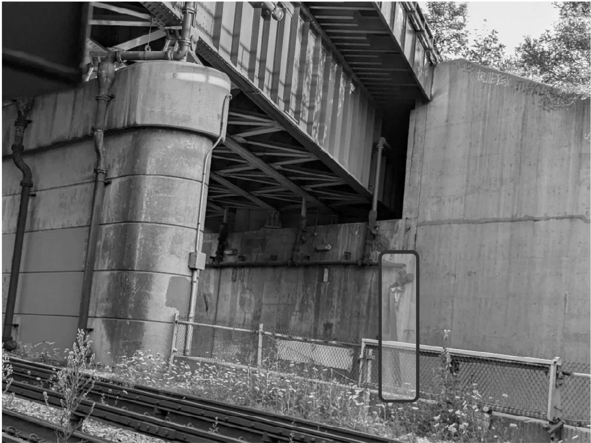
016-0517 PHOTO #1 NORTH ABUTMENT REPAIR 6 INCH CAST IRON PIPE FROM HORIZONTAL TOP SECTION TO ROADWAY SURFACE, 24 FEET
