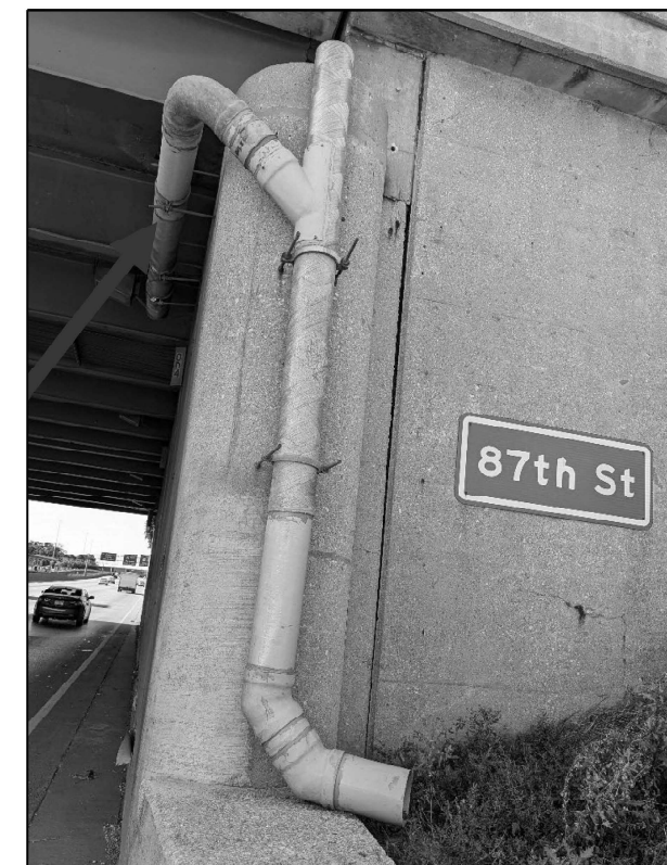
016-1142 PHOTO #1 NORTHWEST CORNER OF THE BRIDGE REPLACE DAMAGED HORIZONTAL RUN, 4 FEET
