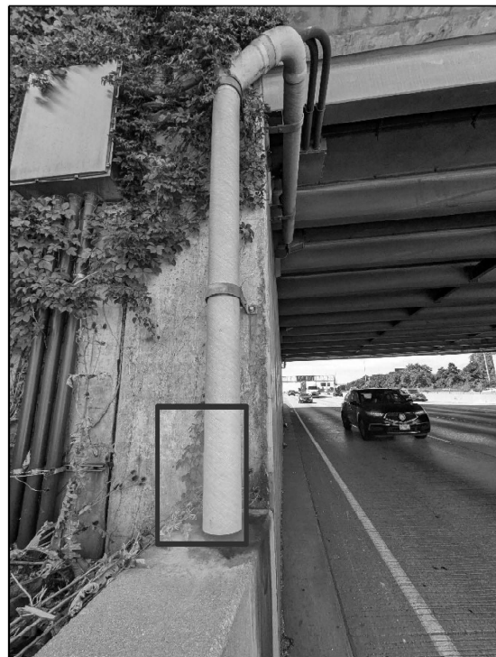
016-1143 PHOTO #4 EAST ABUTMENT - NORTH END ELBOW TO PUSH WATER BEHIND BARRIER, 4 FEET
