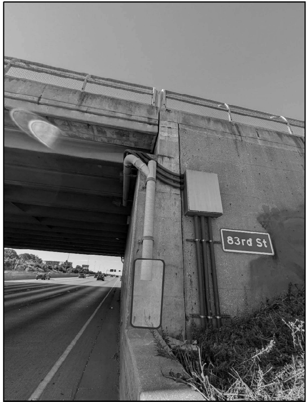
016-1143 PHOTO #1 NORTHWEST CORNER OF BRIDGE REPLACE ELBOW AND PIPE EXTENSION TO MOVE WATER BEHIND BARRIER WALL, 4 FEET
