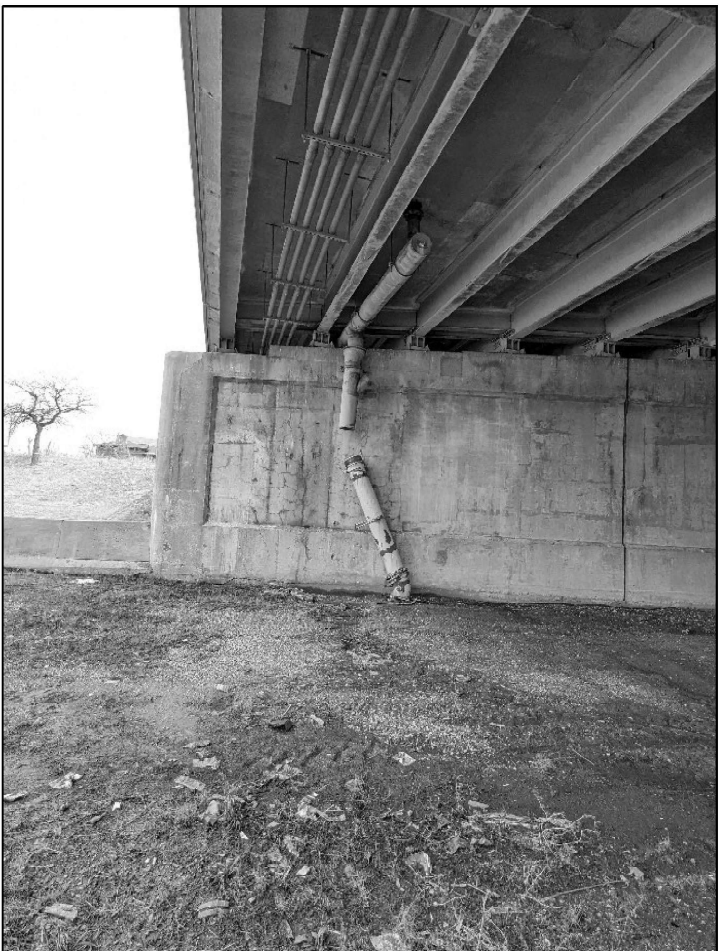
016-0989 PHOTO #2 WEST FACE OF EAST PIER - NORTH PIPE
