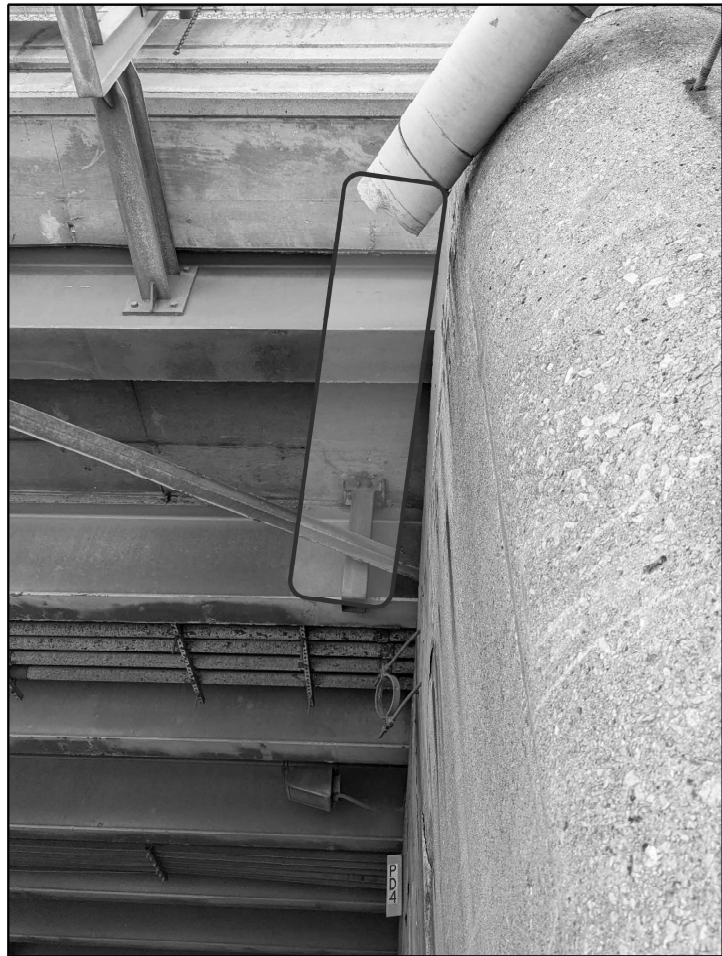
016-1144 PHOTO #1 REPLACE ELBOW AND CONNECTION TO DOWNSPOUT, 8 FEET
