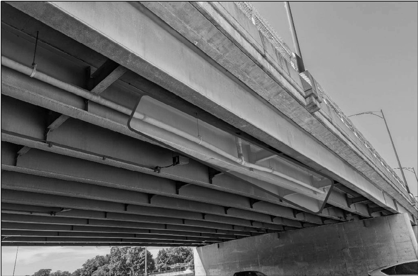
016-2850 PHOTO #2 REPLACE PIPE ON NORTH SIDE OF BRIDGE - OVER NORTHBOUND LANES, 50 FEET
