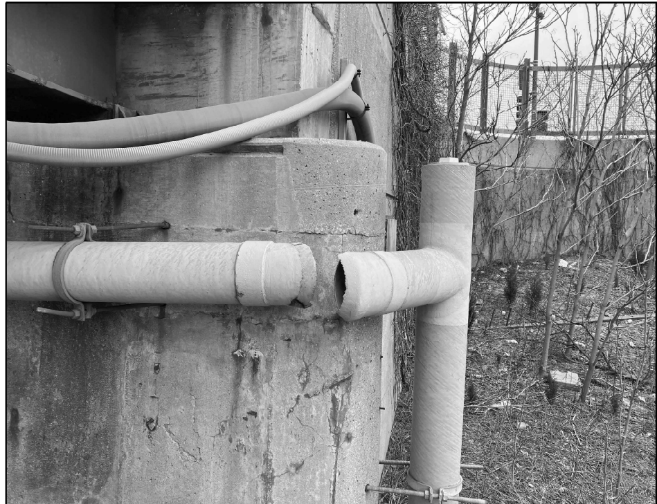
016-0189 PHOTO #2 EAST ABUTMENT DRAINAGE REPLACE 60 DEGREE ELBOW, 2 FEET
