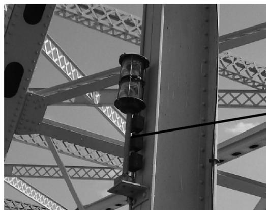
Replace Each White Navigation Light Assembly with LED Navigation Light Assemblies (see Construction Sequence on Sheet S12)
