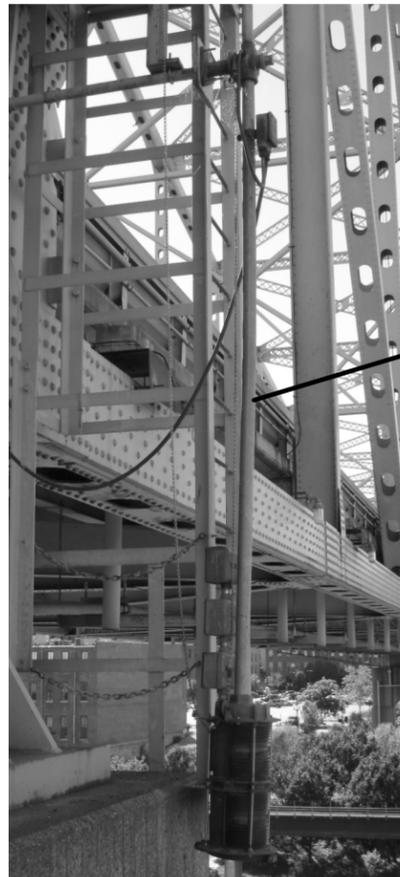
Replace Each Span Navigation Light Assembly with LED Navigation Light Assemblies at Existing Mounting Brackets
