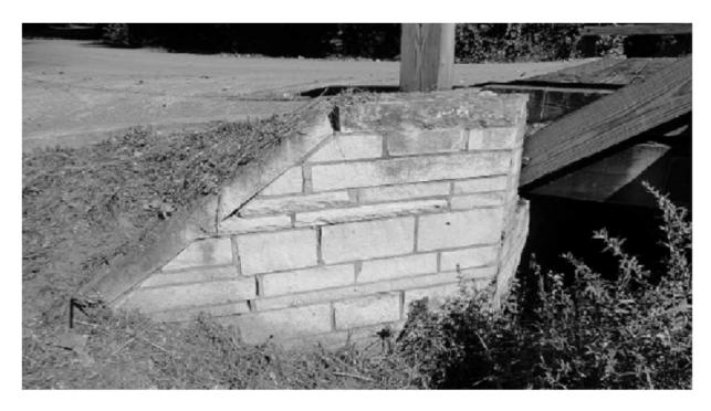
The cost of all the labor, materials and equipment necessary to complete the work as indicated in this Special Provision and the details in the plans shall be included in the contract unit price per Lump Sum for RECONSTRUCT STONE FACING ON WINGWALL.
