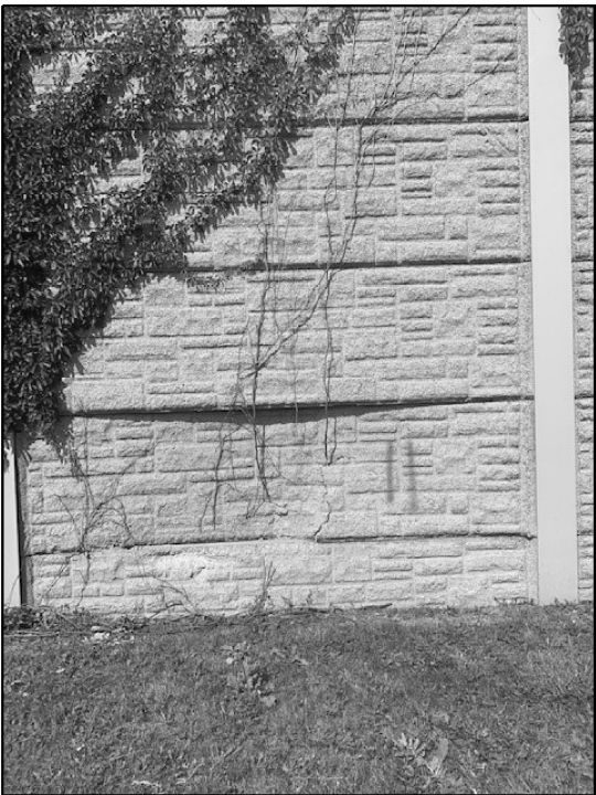
PRECAST CONCRETE WALL REPLACE 3 FT X 12 FT SECTION
