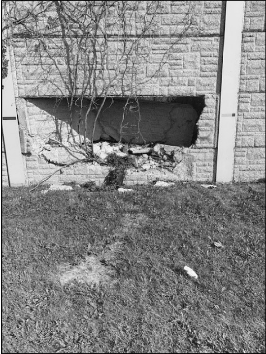
PRECAST CONCRETE WALL REPLACE TWO 3 FT X 12 FT SECTIONS
