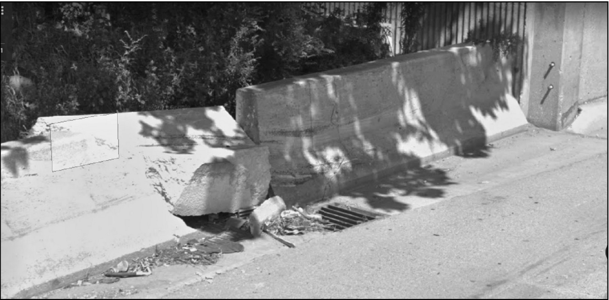
LOCATION 11. FULL DEPTH BARRIER WALL REPAIR REPLACE 6 FT OF PARAPET LOCATED AT I-290 WB AT WEST OF PAULINA AVE. RIGHT SIDE
