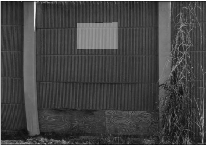
DURISOL TYPE WALL REPLACE 14.5 FT X 3FT PANEL
