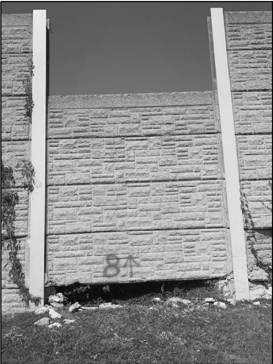
PRECAST CONCRETE WALL REPLACE THREE (3) 3 FT X 12 FT SECTIONS
