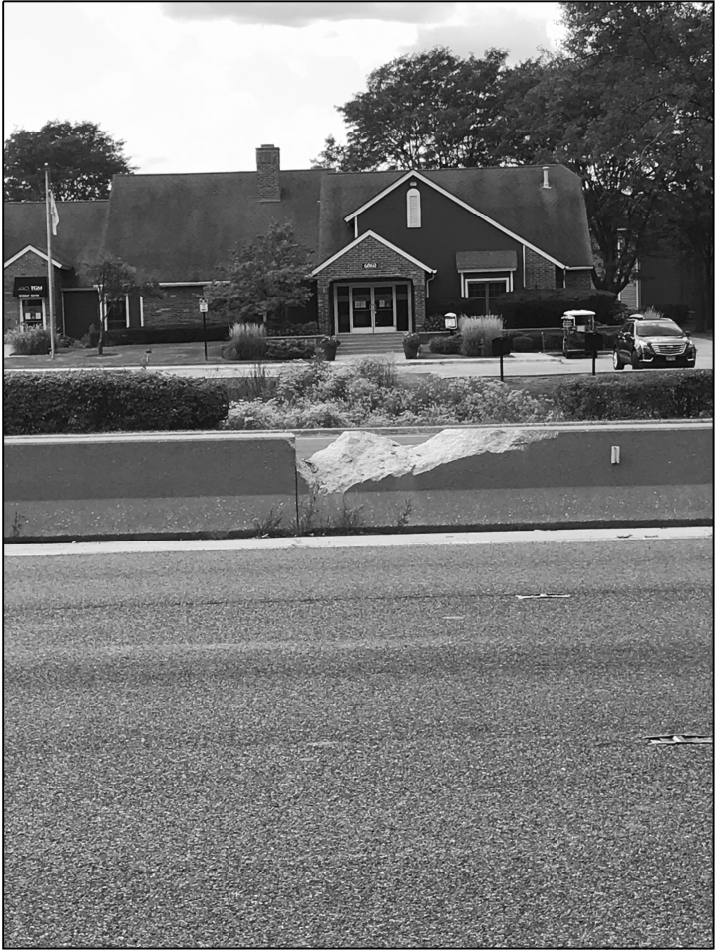
LOCATION 22. PARTIAL DEPTH BARRIER WALL REPAIR REPLACE 8 FT OF PARAPET LOCATED AT ILL 83 MEDIAN BETWEEN 63rd ST AND 55th ST
