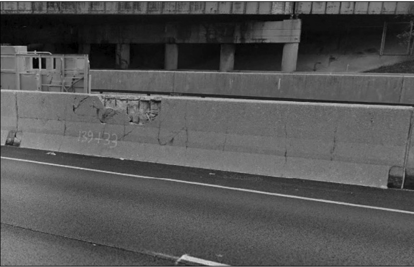
LOCATION 19. FULL DEPTH BARRIER WALL REPAIR REPLACE 8 FT OF PARAPET LOCATED AT I-90/94 NWB AT SOUTH OF FOSTER AVE. LEFT SIDE
