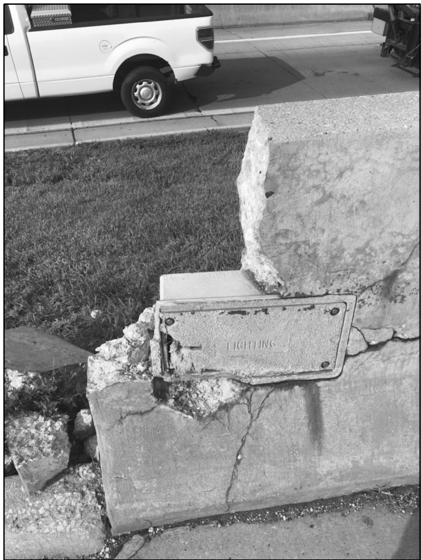
LOCATION 16. FULL DEPTH BARRIER WALL REPAIR REPLACE 2 FT OF PARAPET LOCATED AT I-90/94 SB AT WEBSTER AVE.
