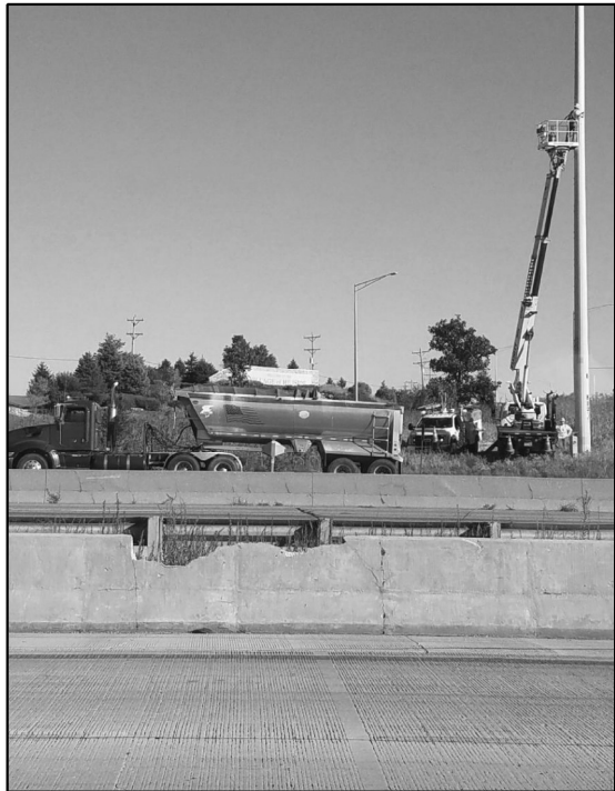
LOCATION 15. FULL DEPTH PARAPET REPAIR REPLACE APPROXIMATELY 7'-11" OF PARAPET LOCATED AT EB WEST OF MANNHEIM RD IN LOCALS LEFT SIDE
