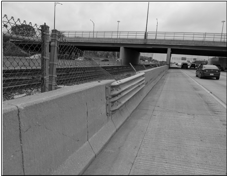
LOCATION 5. HALF DEPTH BARRIER WALL REPAIR REPLACE APPROXIMATELY 16 FT OF BARRIER WALL LOCATED AT NB I-90/94 (DAN RYAN) NORTH OF 76th ST LEFT SIDE CTA WALL
