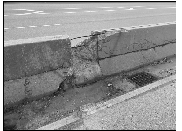
LOCATION 8. FULL DEPTH MEDIAN BARRIER WALL REPAIR REPLACE APPROXIMATELY 5 FT OF PARAPET LOCATED AT 1500 FT SOUTH OF GRAND AVE IN GURNEE
