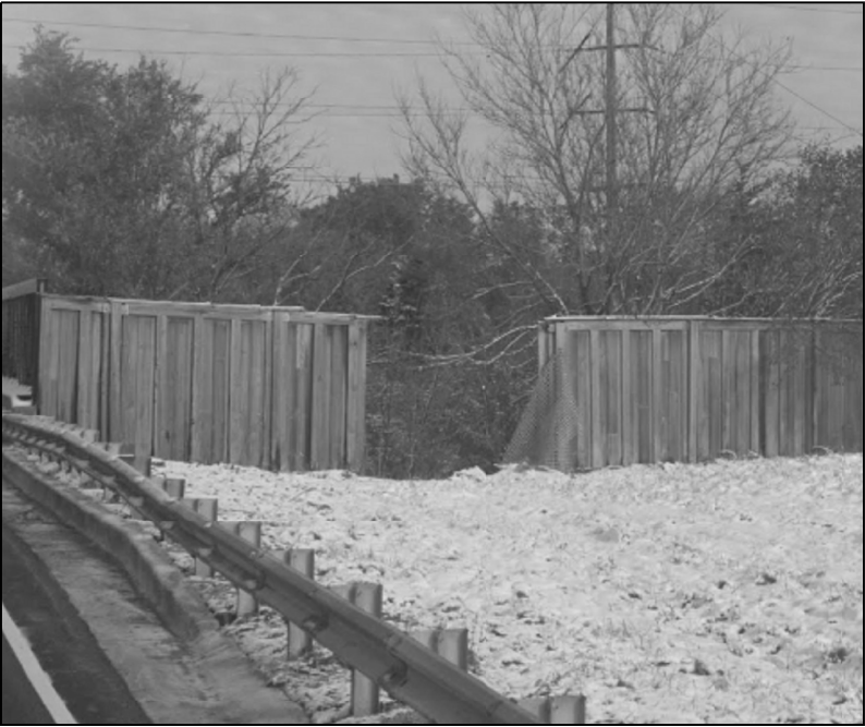
LOC 24. WOOD NOISE WALL REPLACE 15 FT X 8 FT WOOD PANEL
