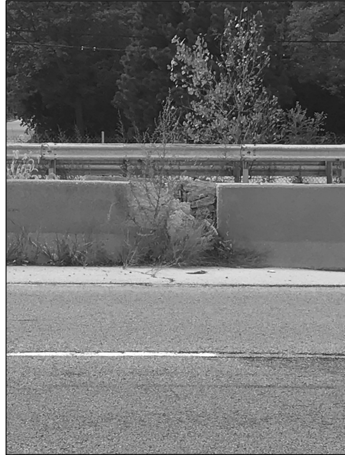
LOCATION 21. FULL DEPTH BARRIER WALL REPAIR REPLACE 13 FT OF PARAPET LOCATED AT ILL 83 MEDIAN BETWEEN RIVERSIDE DR AND IL 38
