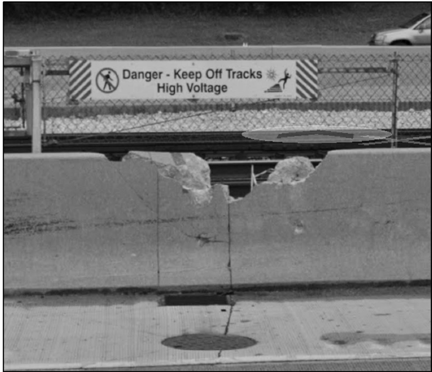
LOCATION 18B. PARTIAL DEPTH BARRIER WALL REPAIR REPLACE 13 FT OF PARAPET LOCATED AT I-90/94 NB AT NORTH OF ADDISON ST. LEFT SIDE
