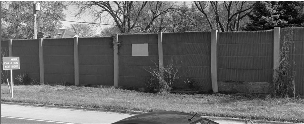
DURISOL TYPE WALL REPLACE 14.5 FT X 3FT PANEL
