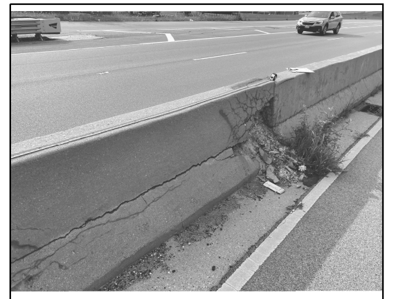
LOCATION 9. FULL DEPTH MEDIAN BARRIER WALL REPAIR REPLACE APPROXIMATELY 5 FT OF PARAPET LOCATED AT 250 FT SOUTH OF GRAND AVE IN GURNEE.
