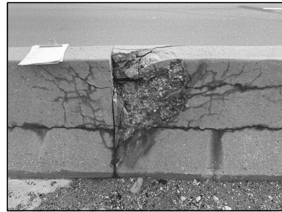
LOCATION 7. FULL DEPTH MEDIAN BARRIER WALL REPAIR REPLACE APPROXIMATELY 5 FT OF PARAPET LOCATED AT 600 FT SOUTH OF GRAND AVE IN GURNEE
