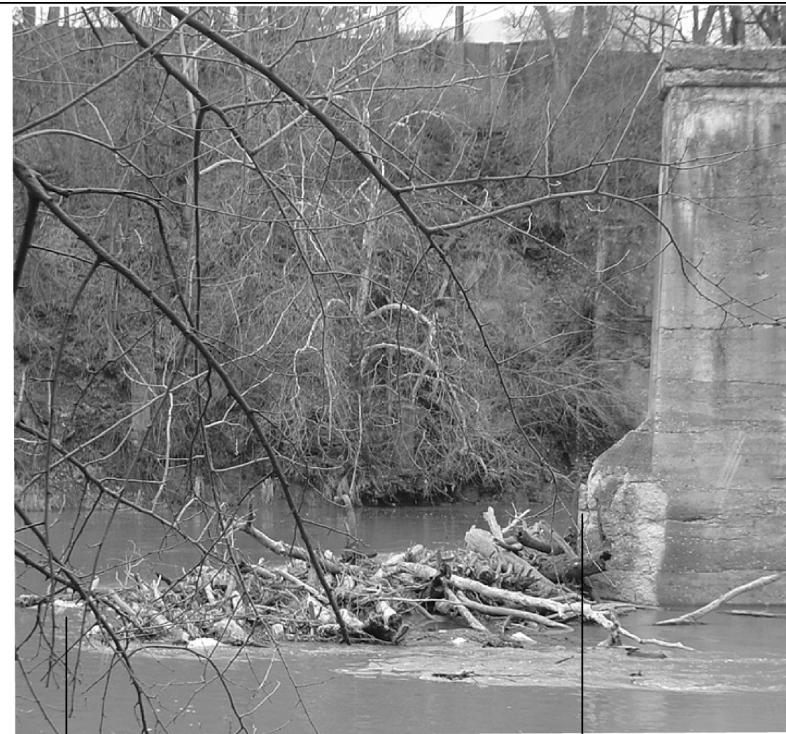
Considered as Organic Debris Removal. Quantity is listed on Sheet 5 in Bill of Materials
