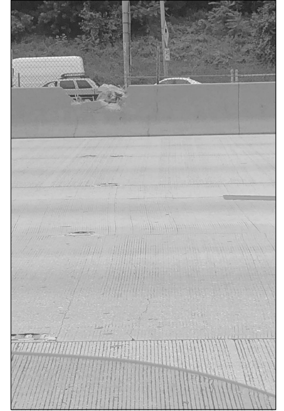
LOC. 18 HALF DEPTH REPAIR REPLACE 10 FT OF BARRIER WALL
