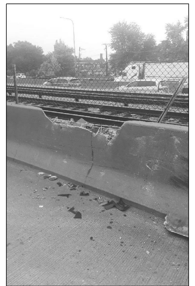
LOC.17 HALF DEPTH REPAIR REPLACE 7 FT OF BARRIER WALL
