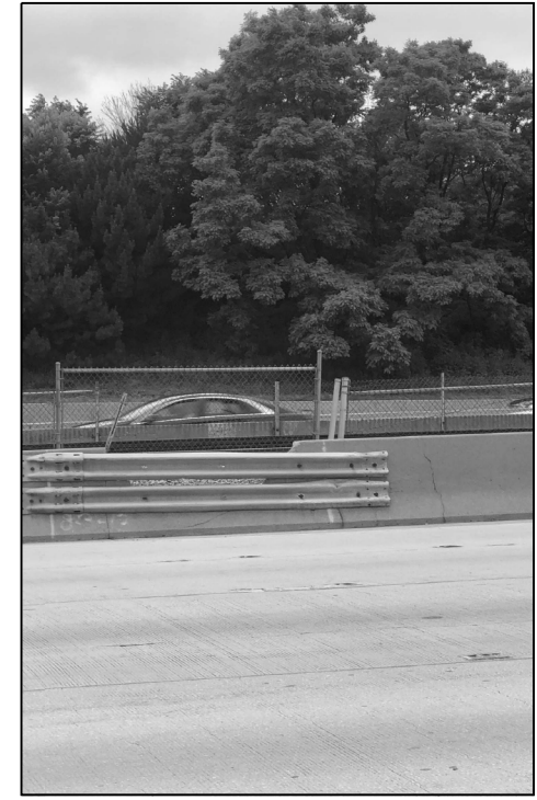
LOC. 19 FULL DEPTH REPAIR REPLACE 11 FT OF BARRIER WALL
