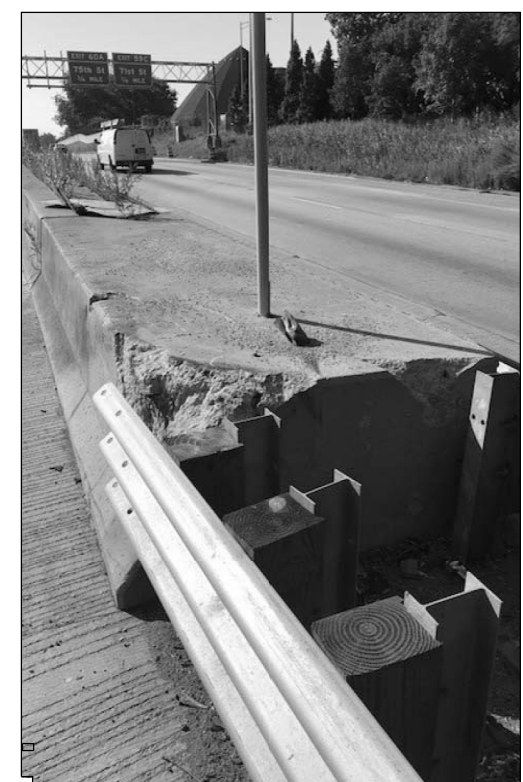
LOC. 20 FULL DEPTH REPAIR REPLACE 17.2 FT OF BARRIER WALL
