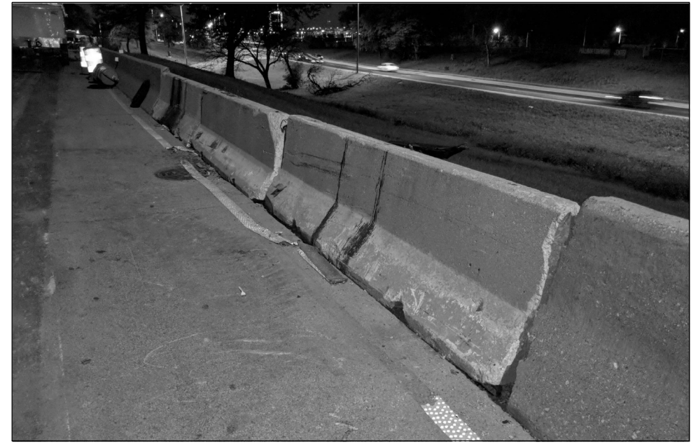
LOC 24. FULL DEPTH REPAIR REPLACE 31 FT OF BARRIER WALL
