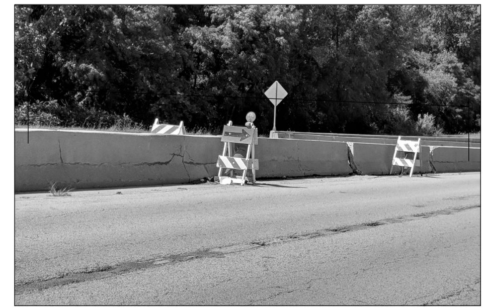
FULL DEPTH REPAIR REPLACE 42 FT OF BARRIER WALL
