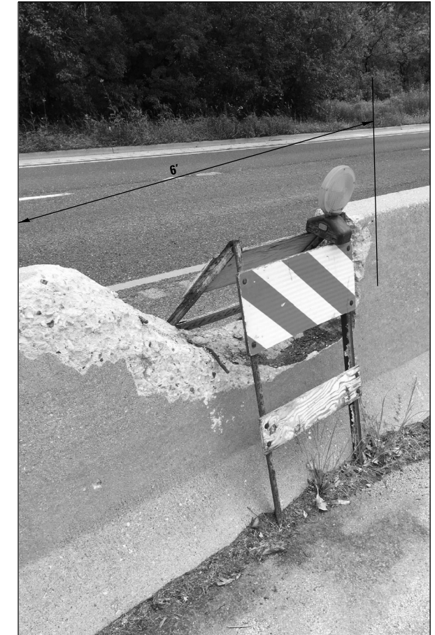
FULL DEPTH REPAIR REPLACE 6 FT OF BARRIER WALL
