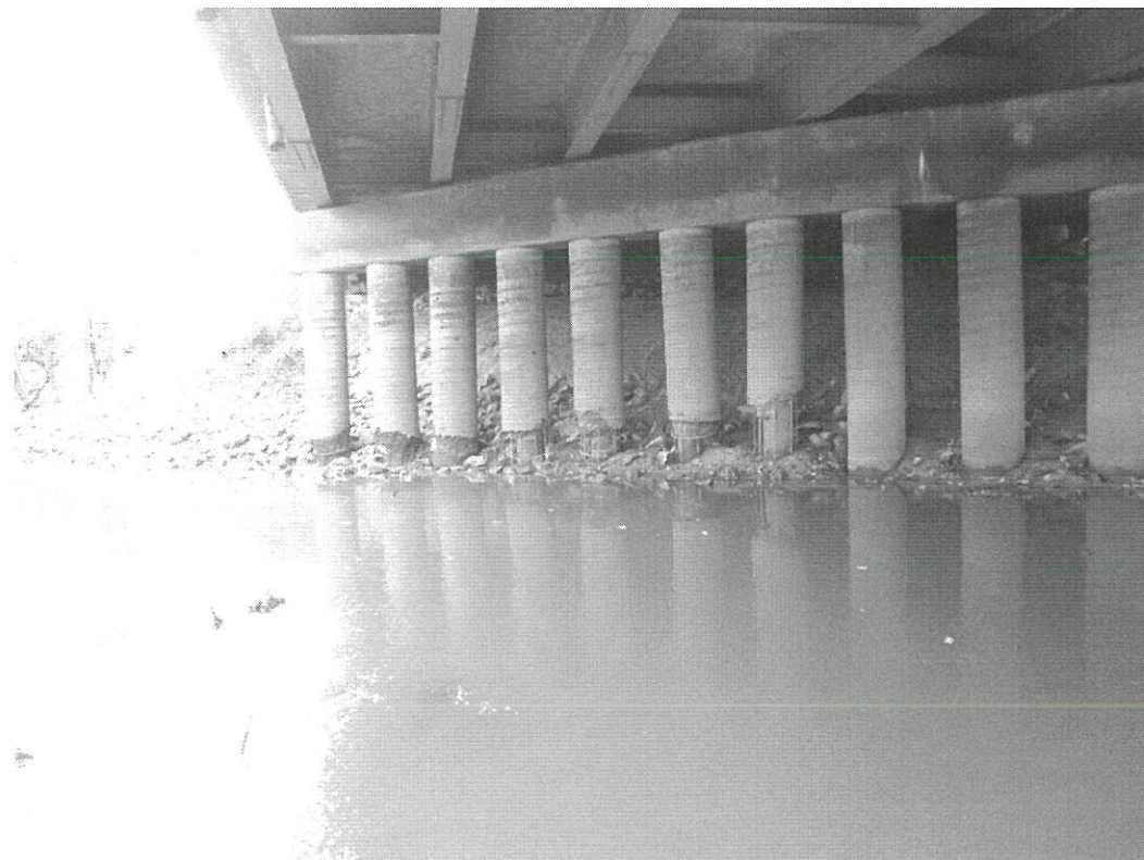
EAST PIER - LOOKING EAST
