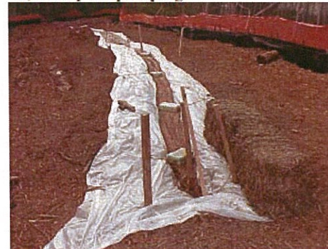
6) Ready for pumping
