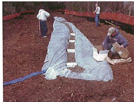
4) Place Floc Logs (upstream end)
