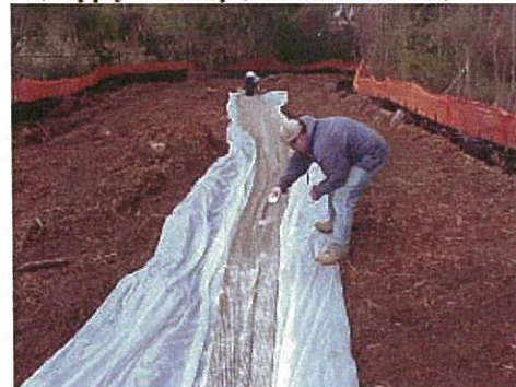
5) Apply Silt Stop (downstream end)
