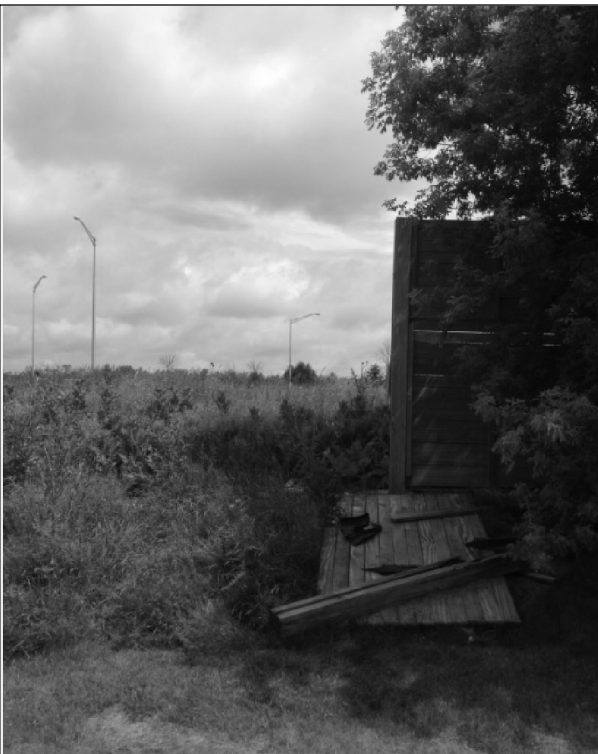
WOOD WALL REPLACE 12 FT X 11 FT OF NOISE WALL
