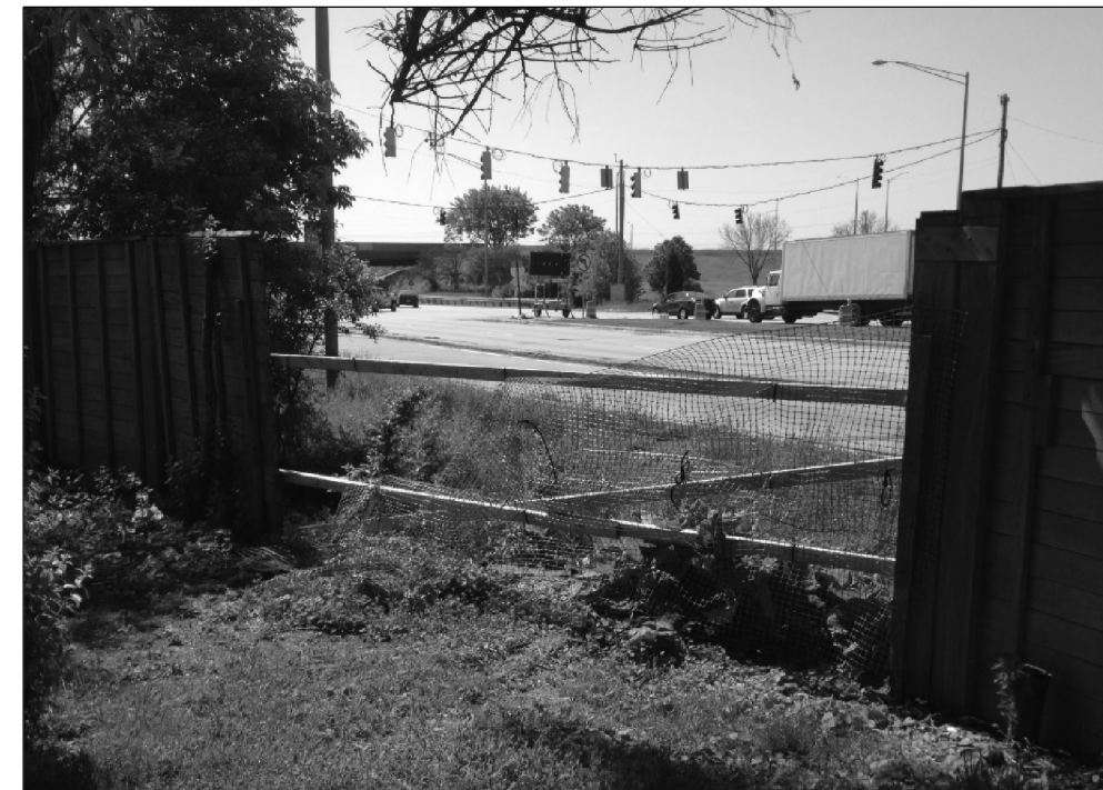
WOOD WALL REPLACE 24 FT X 10 FT OF NOISE WALL
