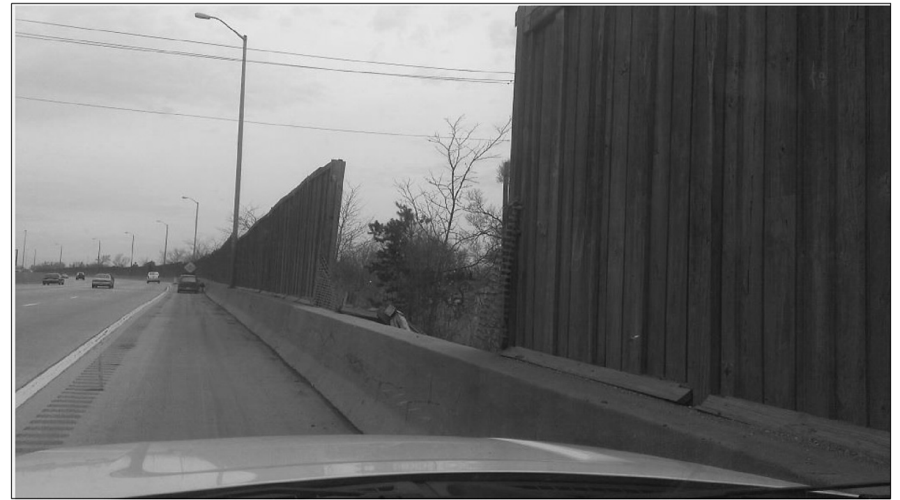
WOOD WALL REPLACE 32 FT X 10 FT OF WOOD WALL
