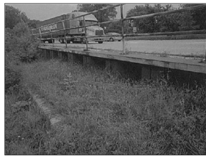
PEDESTRIAN HANDRAIL REPLACE 165 FT OF PIPE HANDRAIL
