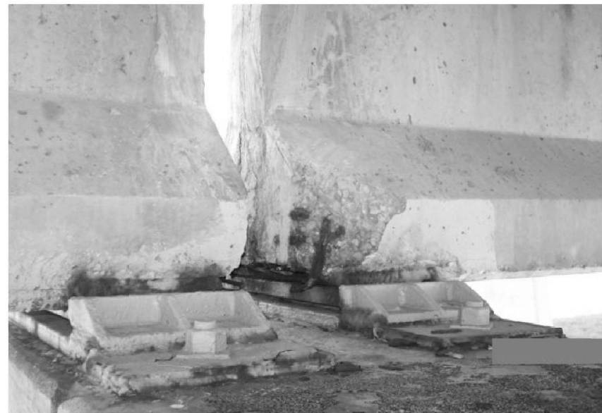
TYPICAL BEARING TO BE CLEANED AND PAINTED.
