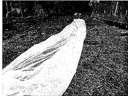
4) Place Flocc Logs (upstream end)
