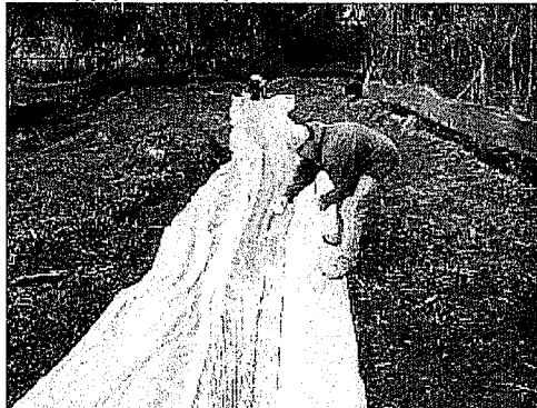
5) Apply Silt Stop (downstream end)
