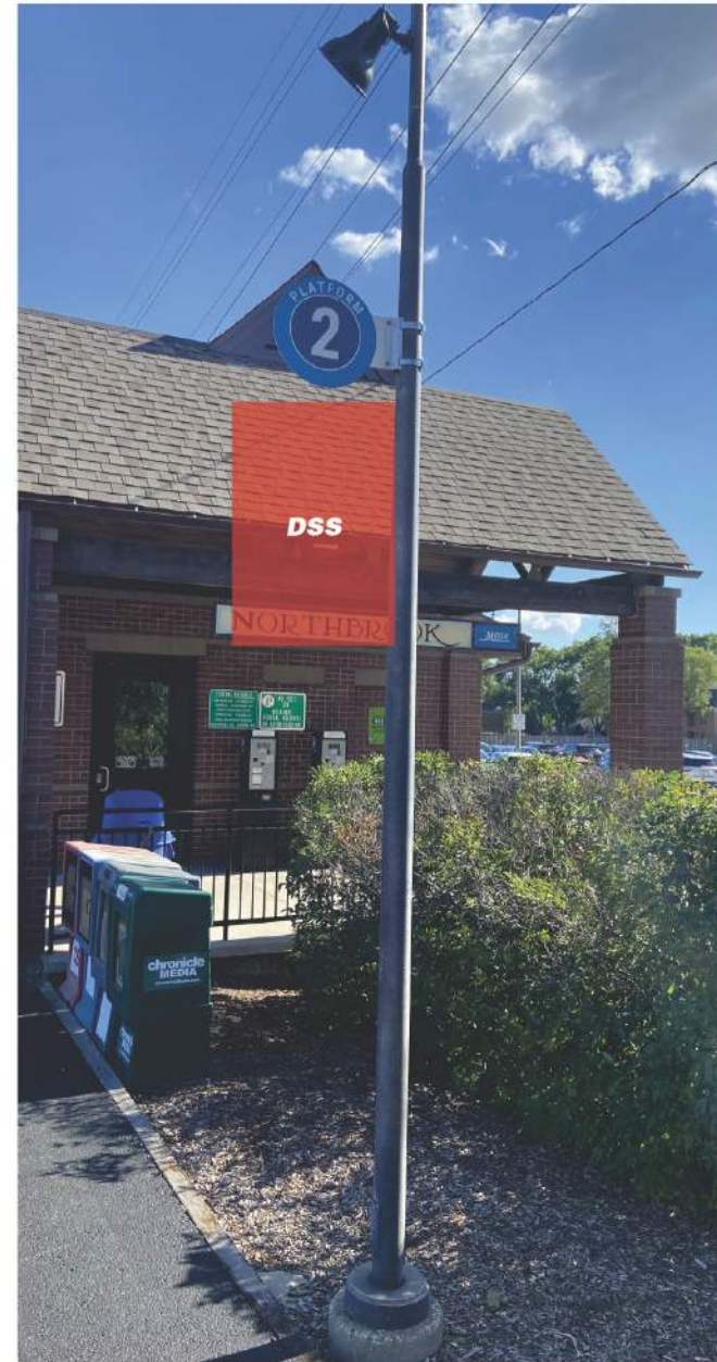
New flag mount mounted on existing light pole.
