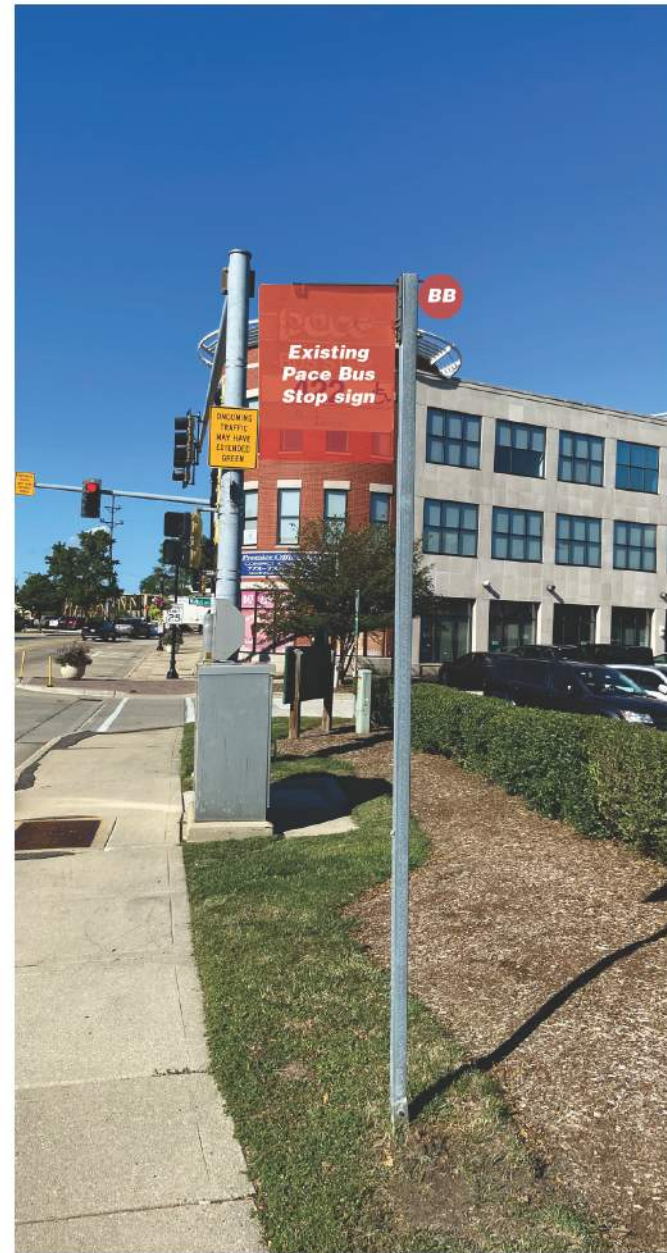
New sign panel mounts to top of existing sign post. Lower existing Pace bus stop sign as needed to accommodate new sign.
