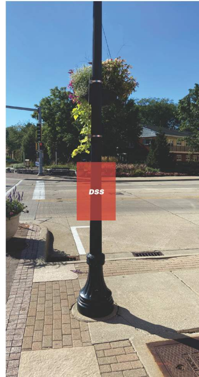
New sign panel mounts to top of existing light pole.
