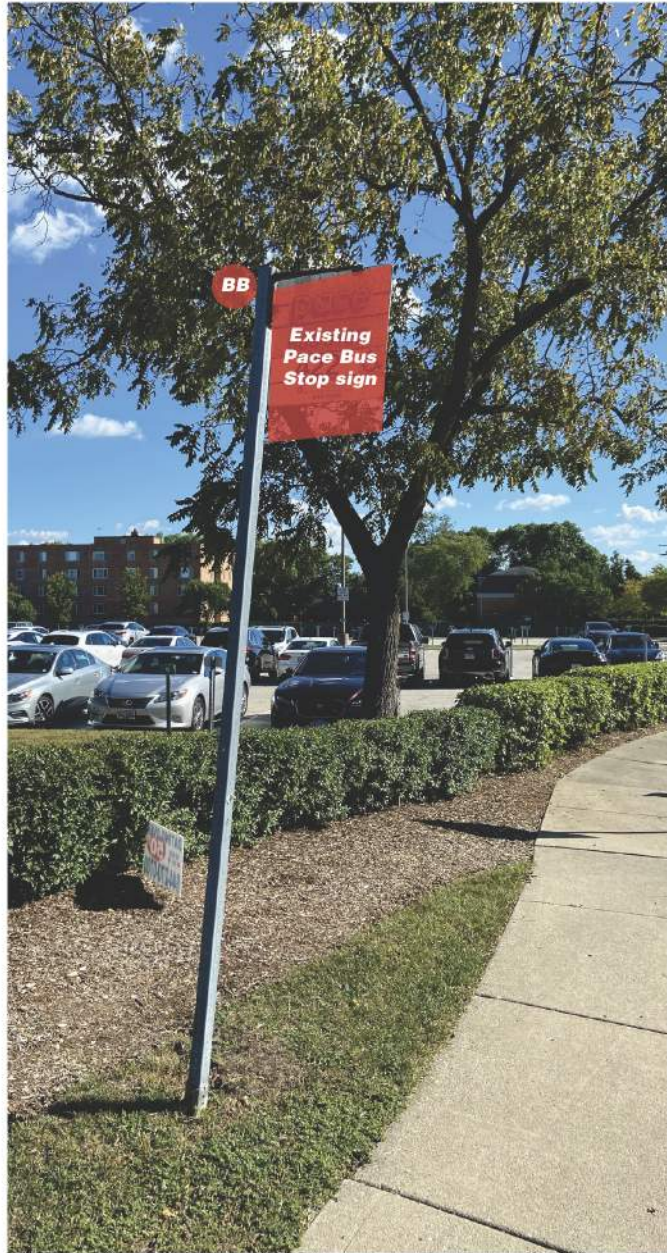
New sign panel mounts to top of existing sign post. Lower existing Pace bus stop sign as needed to accommodate new sign.
