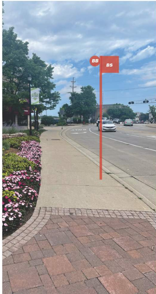
New sign panels mount to new bus stop pole.
