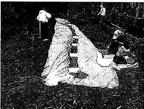
4) Place Flocc Logs (upstream end)
