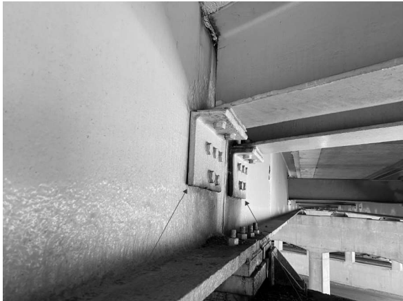
R3 Picture 9: P2; Beam 8 Looking E R7
