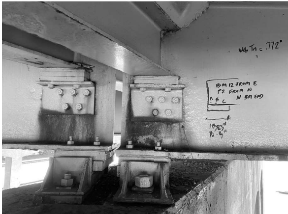
Picture 10: P2; Beam 9 Looking W R4
