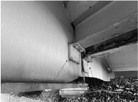
R10 Picture 16: P2; Beam 14 Looking E R16
