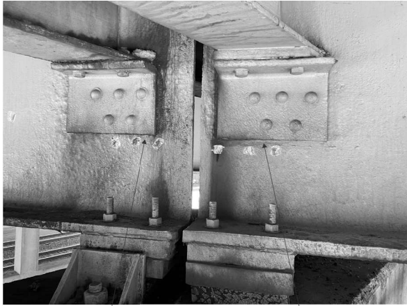
R18 Picture 21: P2; Beam 16 Looking W R12
