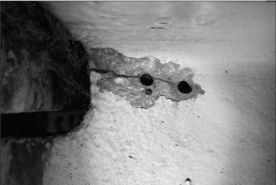
Stringer 1 at Floor Beam FB0' upper web crack that was arrested, no further propagation
