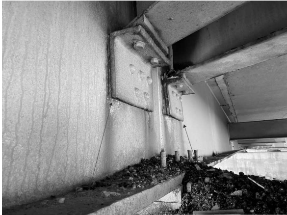
R11 Picture 18: P2; Beam 15 Looking E R17
