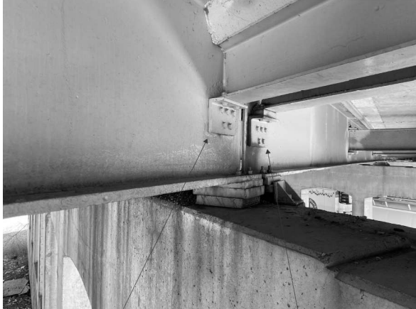
R1 Picture 2: P2; Beam 5 Looking E R5
