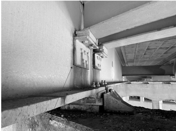
R4 Picture 11: P2; Beam 9 Looking E
