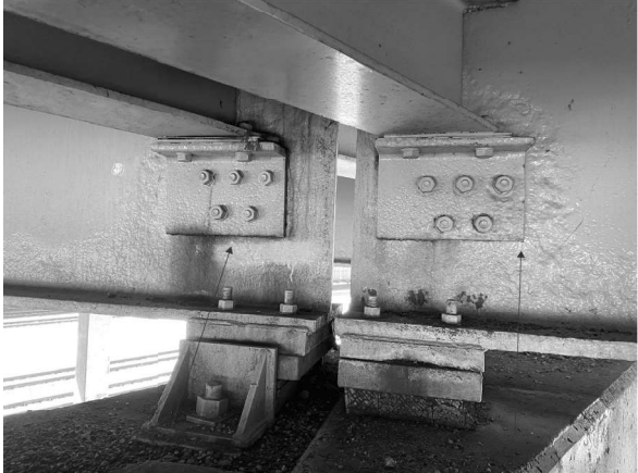
R7 Picture 8: P2; Beam 8 Looking W R3
