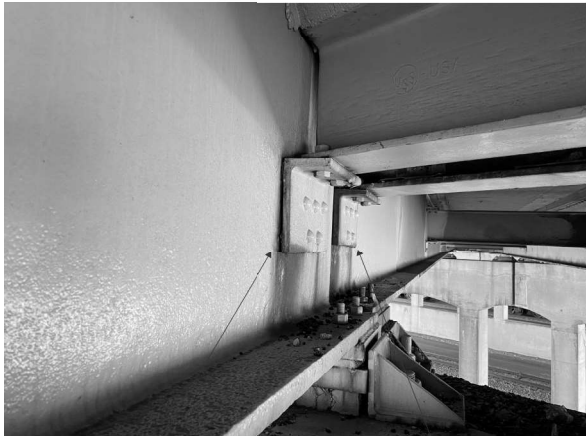
R8 Picture 12: P2; Beam 12 Looking E R14
