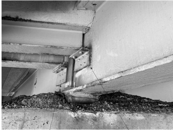
R16 Picture 17: P2; Beam 14 Looking W R10
