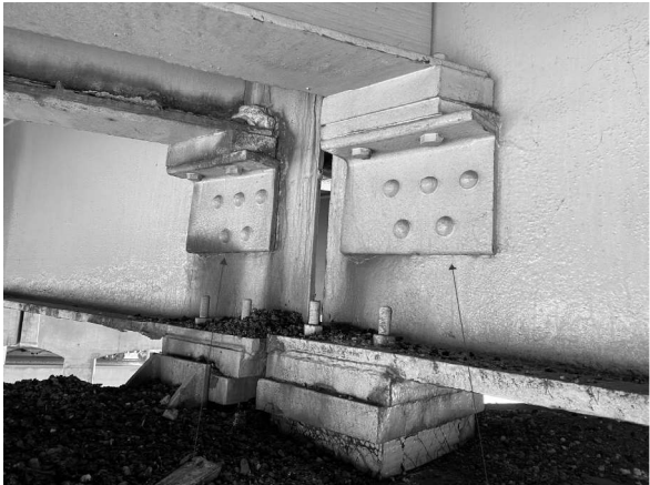
R15 Picture 15: P2; Beam 13 Looking W R9
