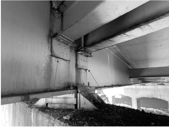
R13 Picture 23: P2; Beam 17 Looking E R19
