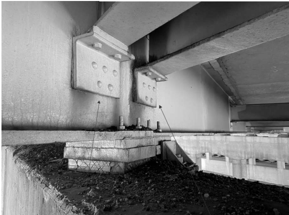
R9 Picture 14: P2; Beam 13 Looking E R15
