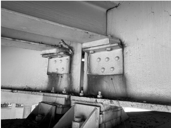
R14 Picture 13: P2; Beam 12 Looking W R8
