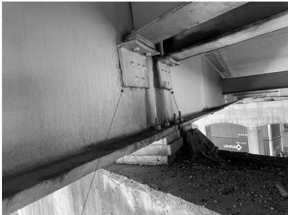
R12 Picture 20: P2; Beam 16 Looking E R18
