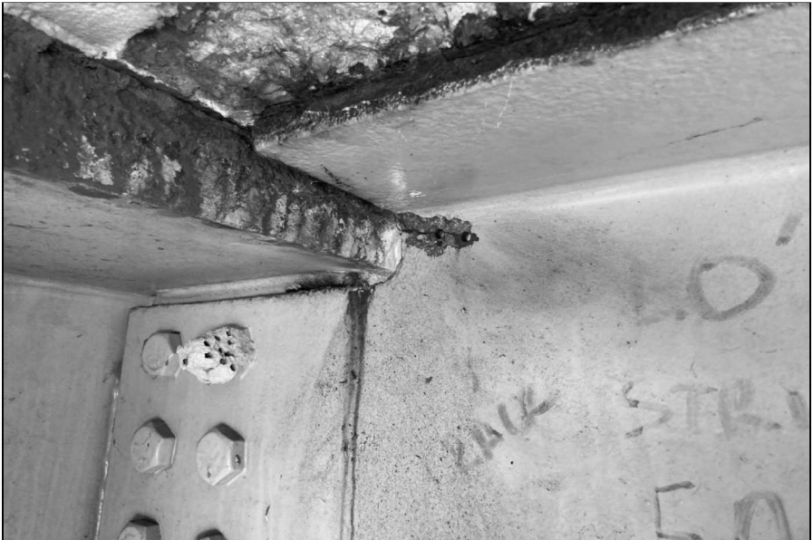
Stringer 1 at Floor Beam FB0' upper web crack
