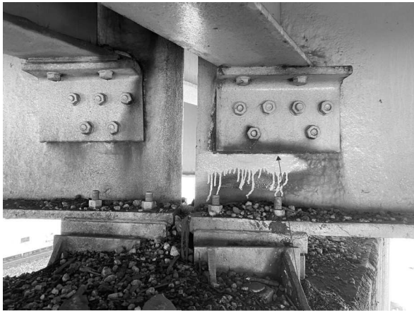
Picture 3: P2; Beam 6 Looking W R2
