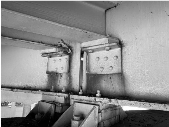
R14 Picture 13: P2; Beam 12 Looking W R8
