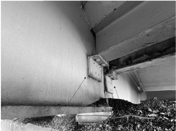
R10 Picture 16: P2; Beam 14 Looking E R16
