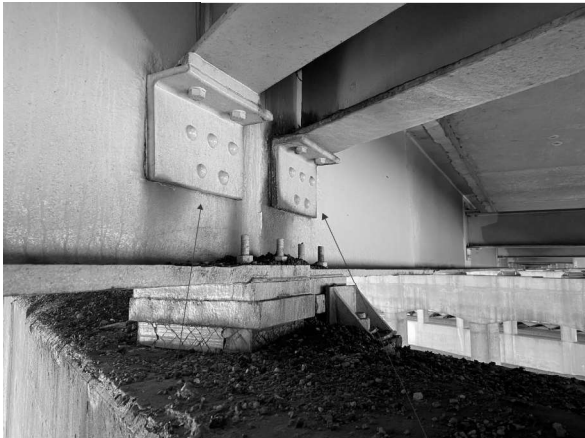
R9 Picture 14: P2; Beam 13 Looking E R15
