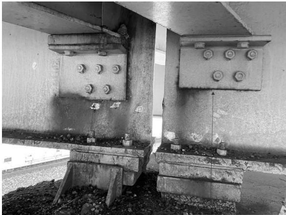
R5 Picture 1: P2; Beam 5 Looking W R1
