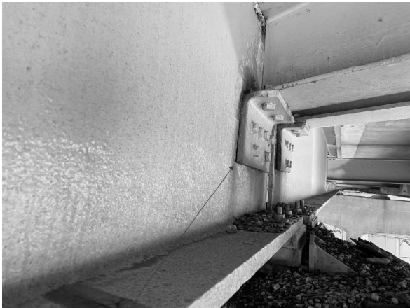
R2 Picture 5: P2; Beam 6 Looking E
