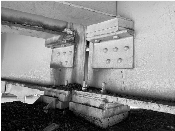
R15 Picture 15: P2; Beam 13 Looking W R9
