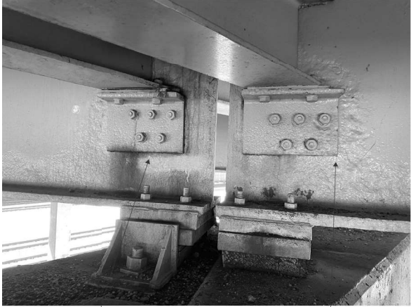
R7 Picture 8: P2; Beam 8 Looking W R3
