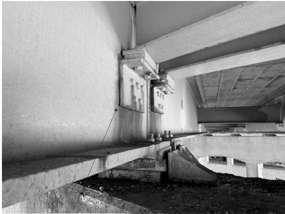
R4 Picture 11: P2; Beam 9 Looking E
