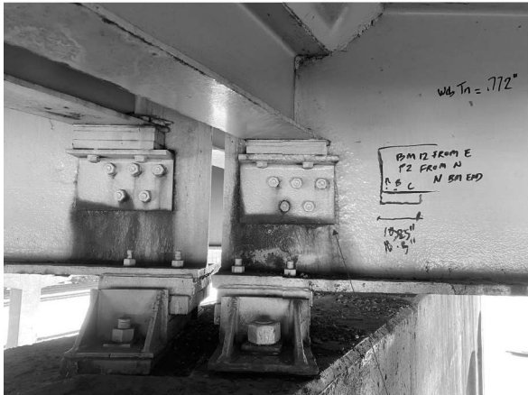
Picture 10: P2; Beam 9 Looking W R4
