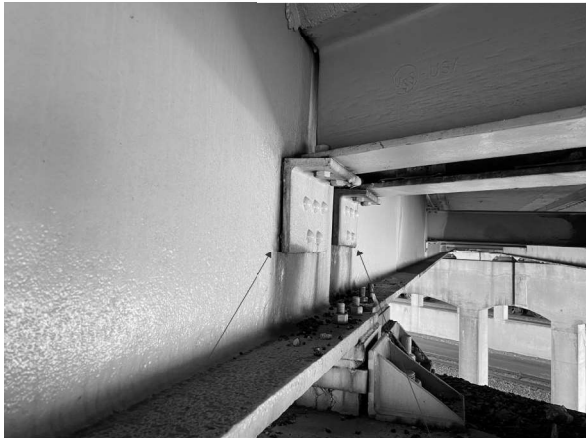
R8 Picture 12: P2; Beam 12 Looking E R14
