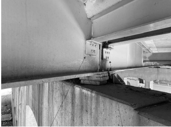
R1 Picture 2: P2; Beam 5 Looking E R5
