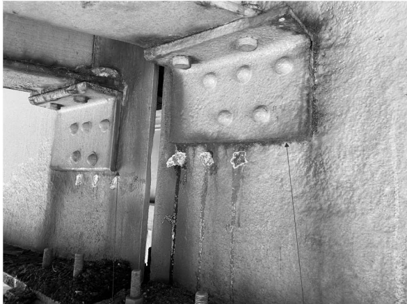
R19 Picture 22: P2; Beam 17 Looking W R13
