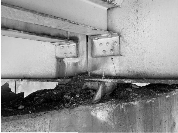
R17 Picture 19: P2; Beam 15 Looking W R11
