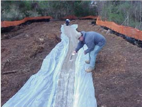
5) Apply Silt Stop (downstream end)
