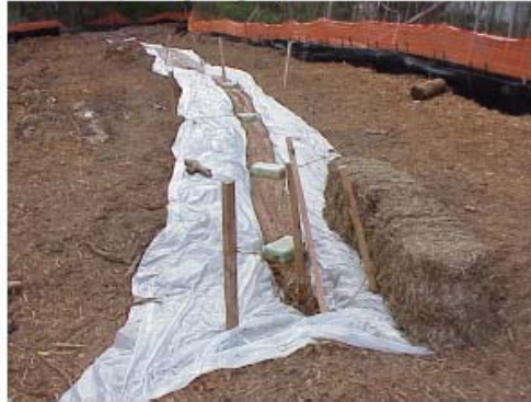
6) Ready for pumping
