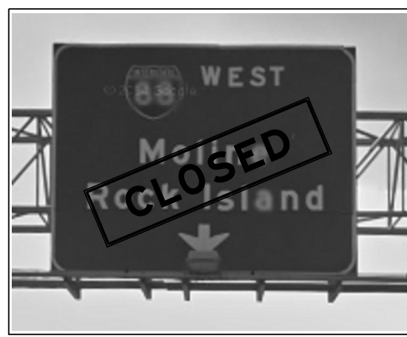
INSTALL CLOSED SIGN ON OVERHEAD SIGN
