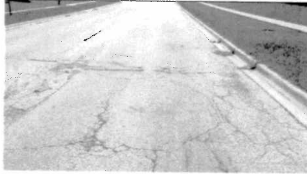
Picture facing West
