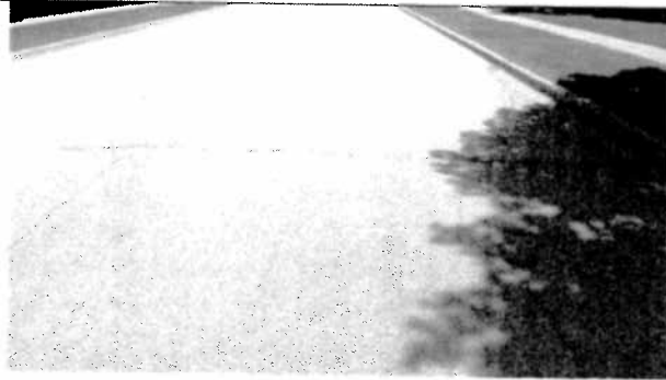
Picture facing East
