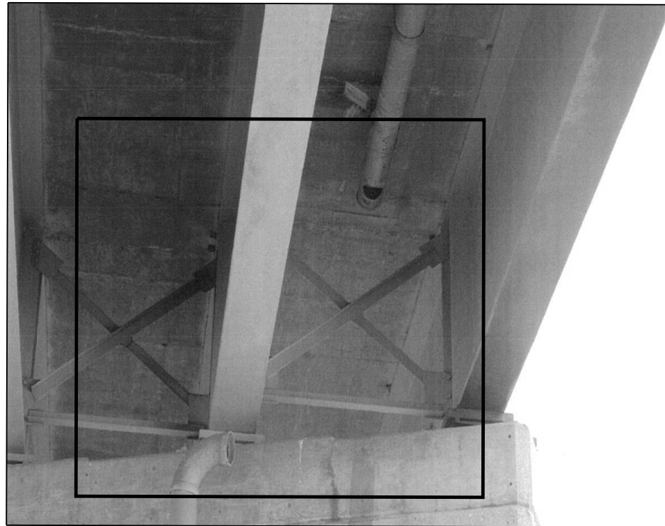
016-0908 PHOTO #1 PIER 1 _ EAST FACE NORTH END
