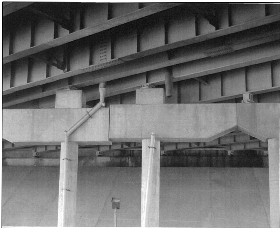
016-0004 AND 016-0005 PHOTO #2 PIER 3 _ WEST FACE
