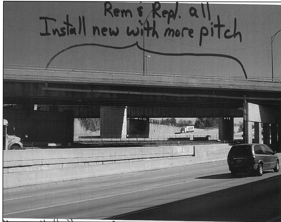
016-1007 PHOTO #1 SECTION OVER DAN RYAN SB EXPRESS LANES _ LOOKING EAST
