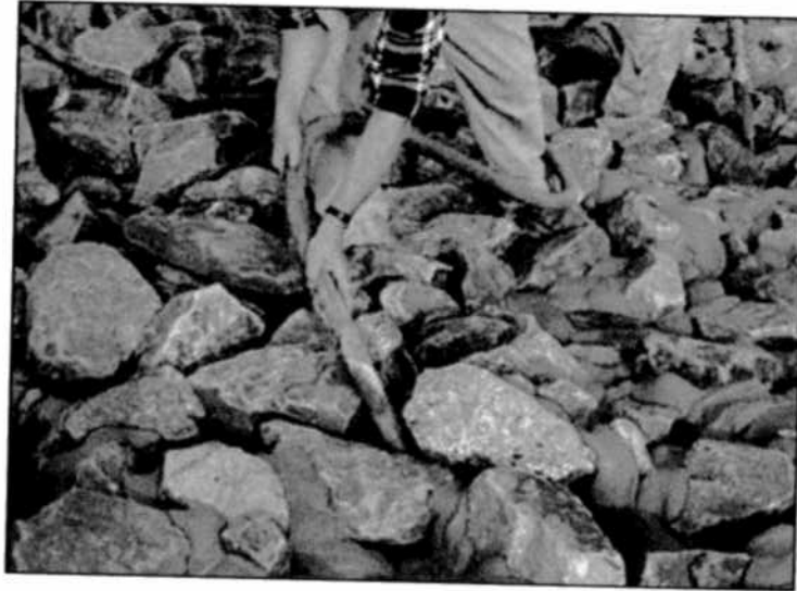
Figure 2: Grout placement by hand
