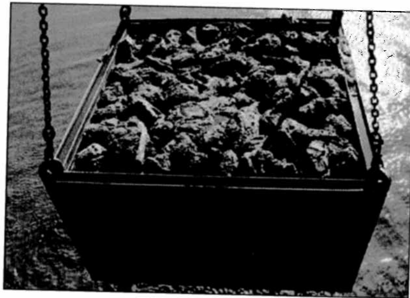
Figure 3: Test box used during underwater grout placement.
