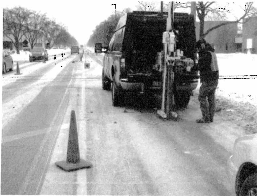
Geoprobe drilling SB-5
