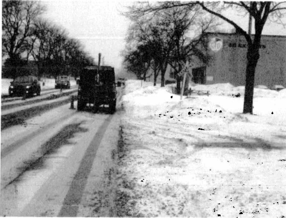
Geoprobe drilling SB-2 on west side of Lively Blvd., view facing south along Lively Blvd.
