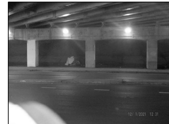
EXISTING LIGHTING: PIER 2 (Looking Northwest)
