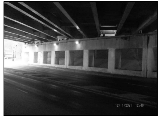
EXISTING LIGHTING: PIER 1 (Looking Northwest)
