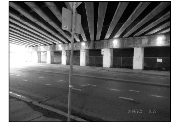
EXISTING LIGHTING PIER 24 (Looking Northwest)
