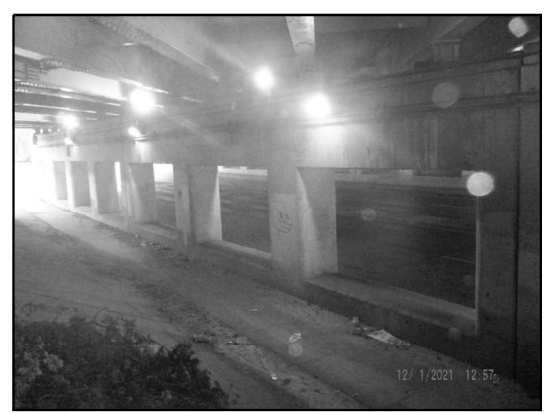
EXISTING LIGHTING: PIER 2 (Looking Northeast)
