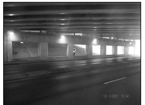
EXISTING LIGHTING: PIER 2 (Looking Southeast)
