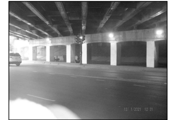
EXISTING LIGHTING: PIER 2 (Looking Northeast)
