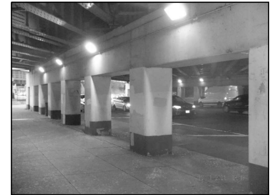
EXISTING LIGHTING: PIER 2 (Looking North)
