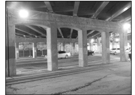
EXISTING LIGHTING: PIER 1 (Looking Northwest)
