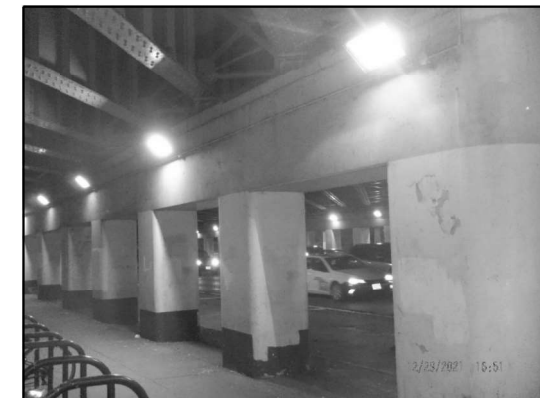
EXISTING LIGHTING: PIER 2 (Looking Northeast)
