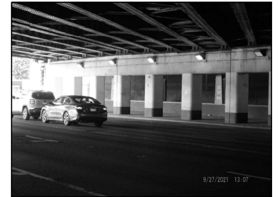
EXISTING LIGHTING: PIER 1 (Looking Northwest)
