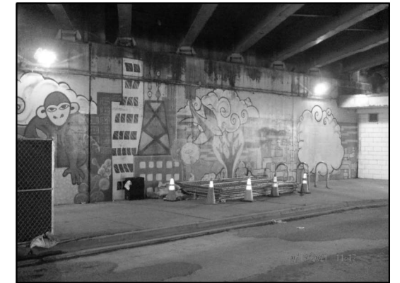
EXISTING LIGHTING: WEST ABUTMENT (Looking Northwest)
