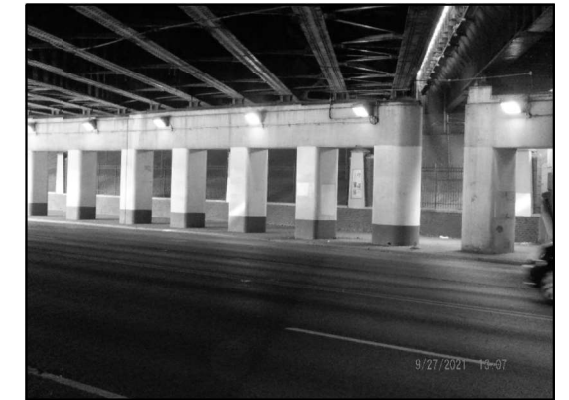
EXISTING LIGHTING: PIER 1 (Looking Northwest)
