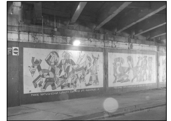
EXISTING LIGHTING: EAST ABUTMENT (Looking Southeast)
