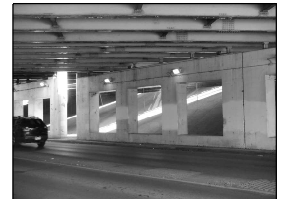
EXISTING LIGHTING: PIER 2 (Looking Southeast)
