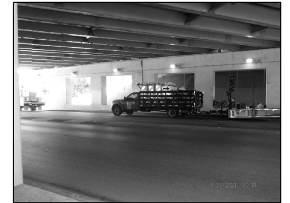
EXISTING LIGHTING: PIER 1 (Looking Southwest)
