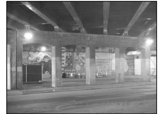
EXISTING LIGHTING: PIER 2 (Looking Northwest)
