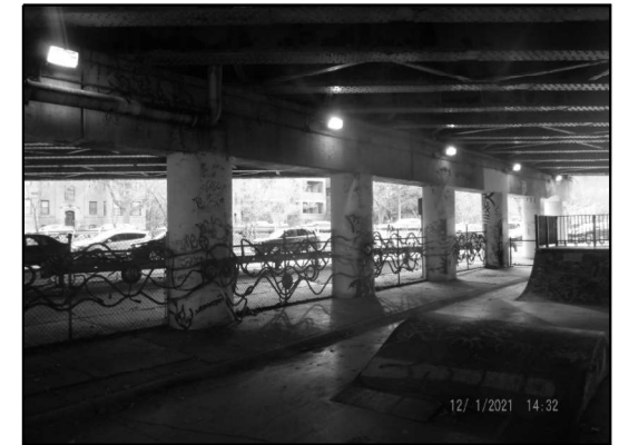
EXISTING LIGHTING: PIER 2 (Looking Northwest)
