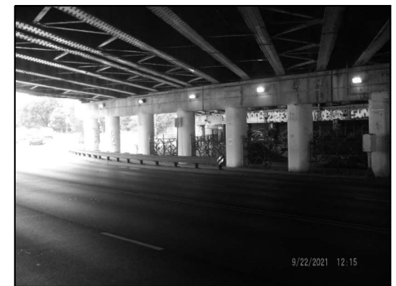
EXISTING LIGHTING: PIER 2 (Looking Northwest)
