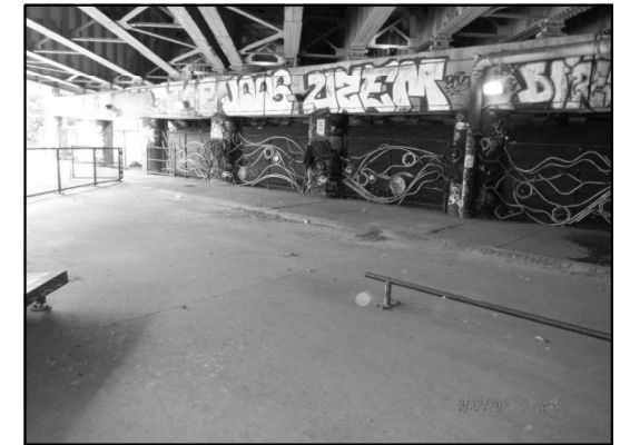
EXISTING LIGHTING: PIER 1 (Looking Northwest)
