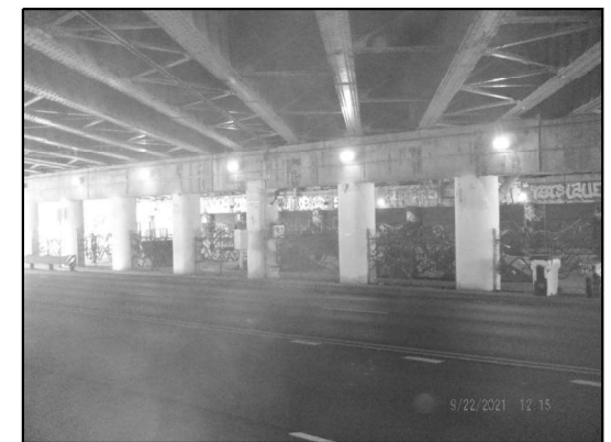
EXISTING LIGHTING: PIER 2 (Looking Northwest)
