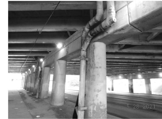
EXISTING LIGHTING: PIER 1 (Looking Northeast)
