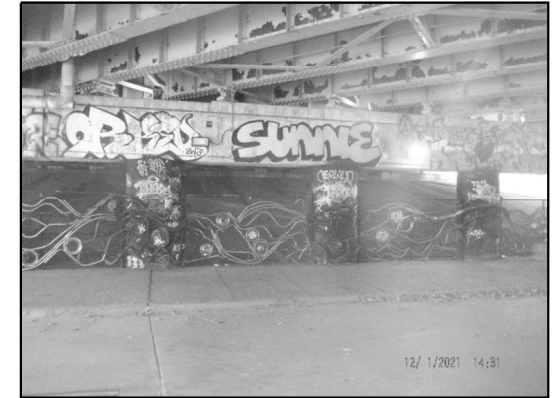
EXISTING LIGHTING: PIER 1 (Looking Northeast)
