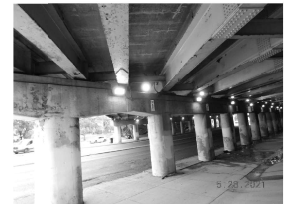
EXISTING LIGHTING: PIER 2 (Looking Northwest)
