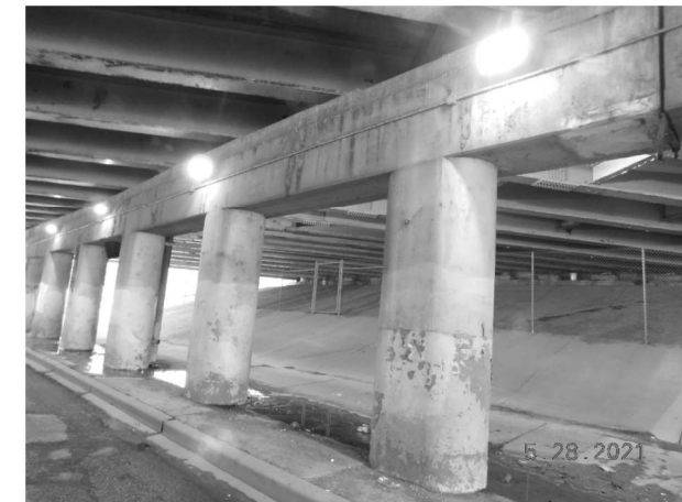
EXISTING LIGHTING: PIER 2 (Looking Northeast)
