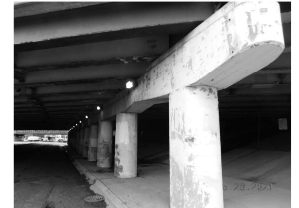
EXISTING LIGHTING: PIER 2 (Looking Northeast)
