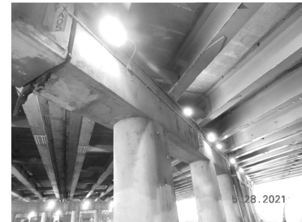
EXISTING LIGHTING: PIER 2 (Looking Northwest)
