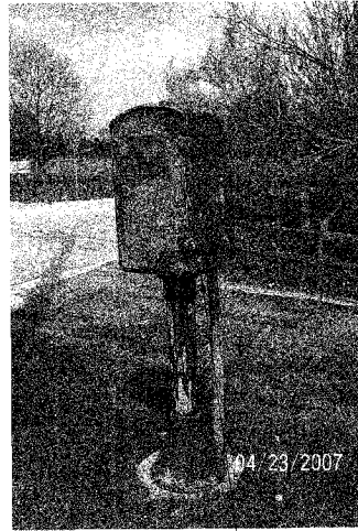
1 EXISTING PEDESTAL MOUNTED CONTROLLER NOT TO SCALE
