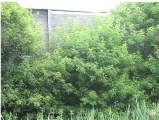
Photo 3. Missing Top Plank (NAW 2)
