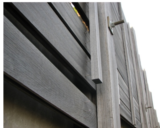
Photos 7 and 8. Loose Planks near South Abutment of SN 022-0137 (NAW 3)
