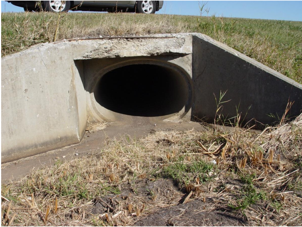
Thorndale Avenue Upstream Face
