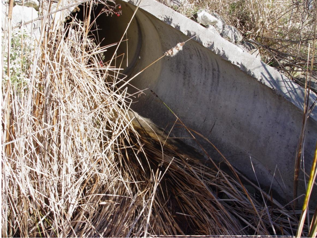
Elgin O'Hare Expressway (West) Upstream Face
