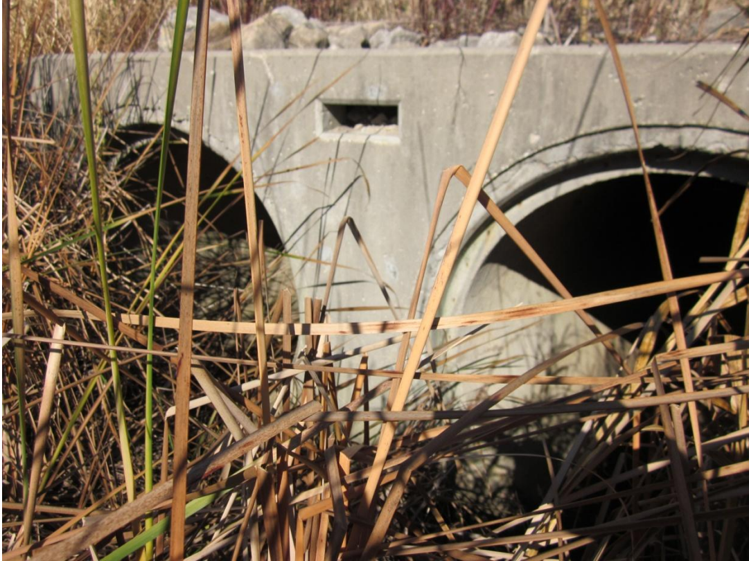
I-290 Ramp Upstream Face
