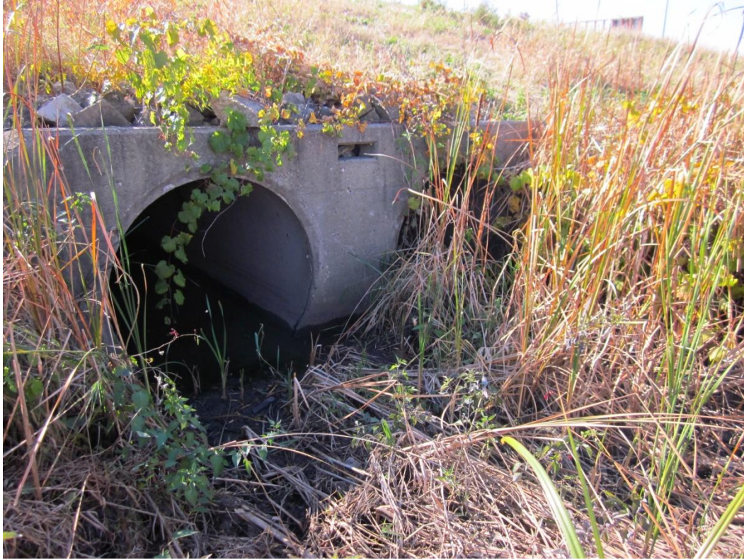
Elgin O'Hare Expressway (East) Downstream Face
