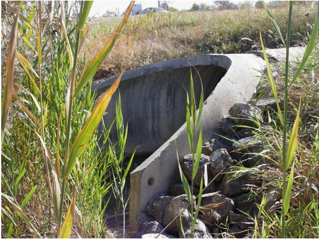
Elgin O'Hare Expressway (West) Downstream Face
