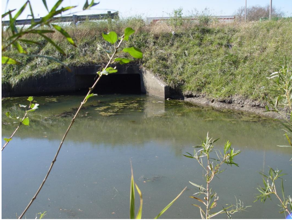
Illinois Route 290 Downstream Face
