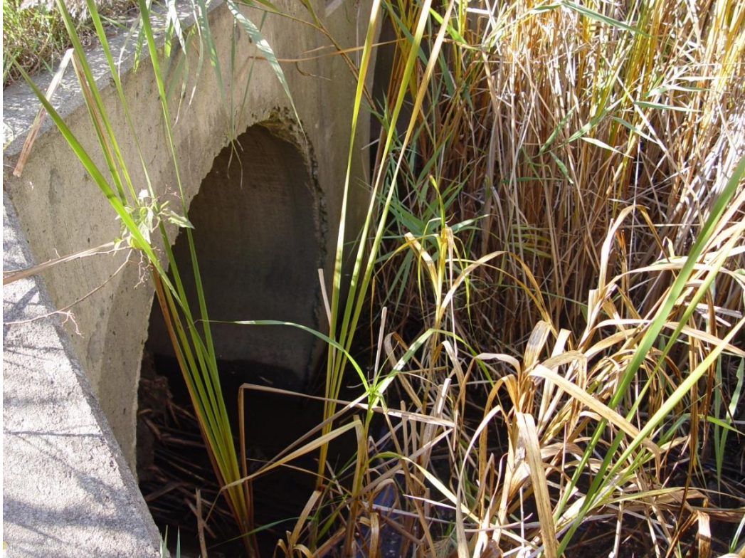
I-290 Ramp Downstream Face
