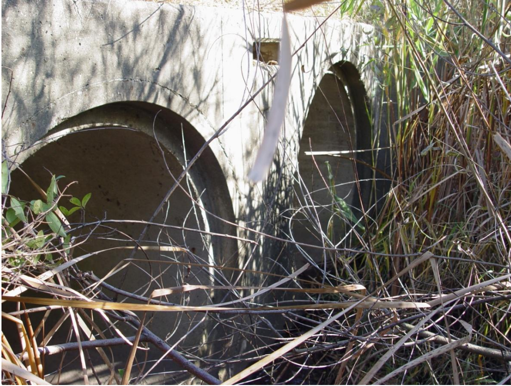
Elgin O'Hare Expressway (East) Upstream Face
